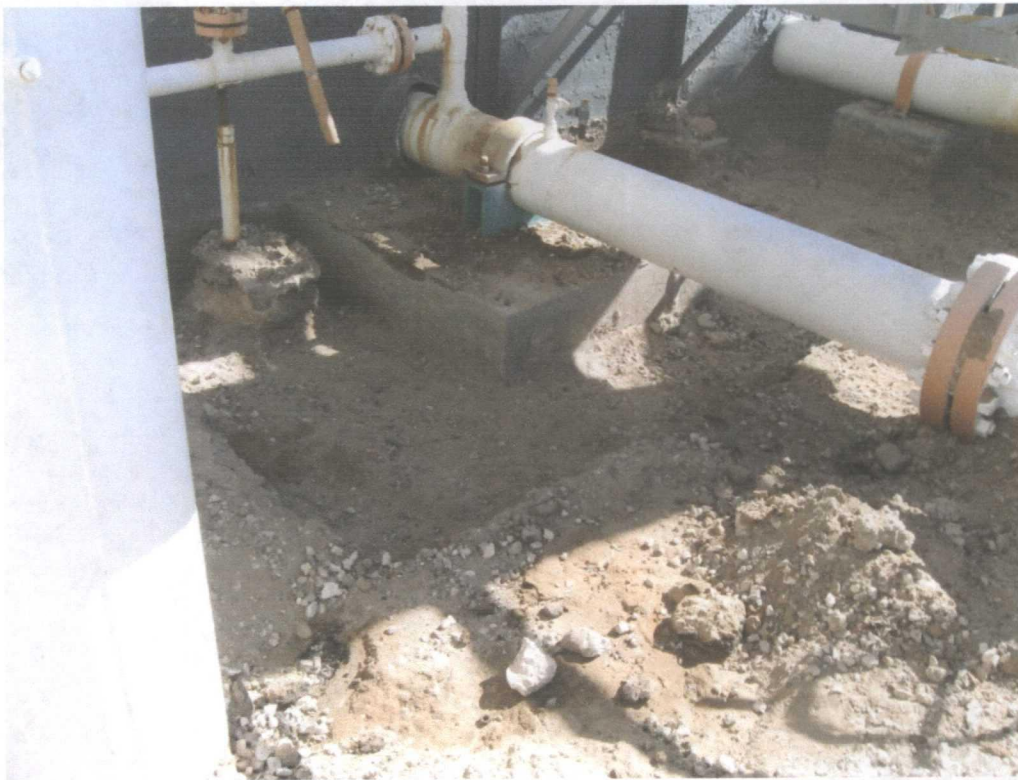
Photo 8 - Compressor area 13 Excavation looking east/northeast
