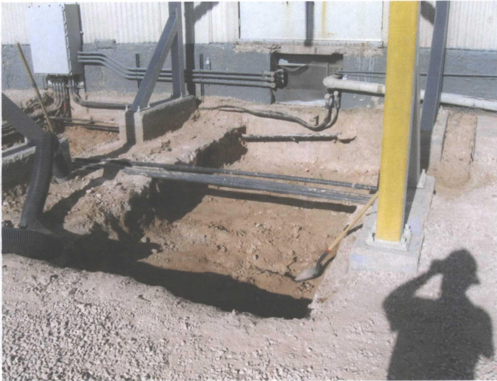
Photo 3 - Compressor area 8 excavation looking west at north half of excavation
