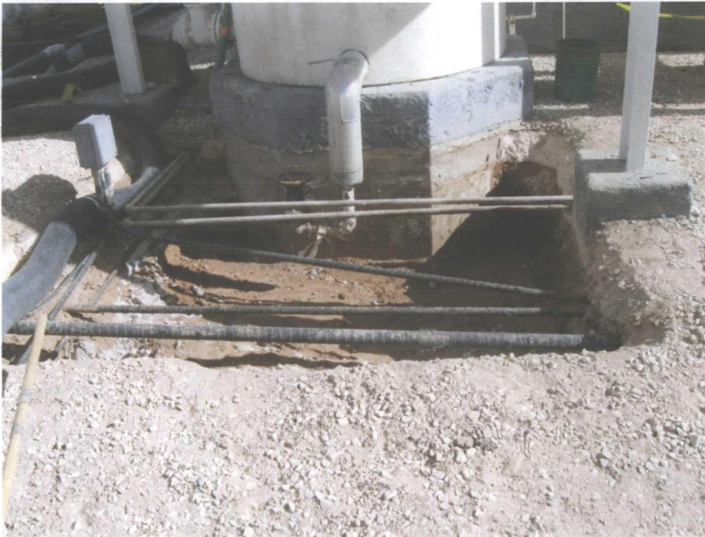
Photo 13 - Partial excavation at Jacket Water Tank
