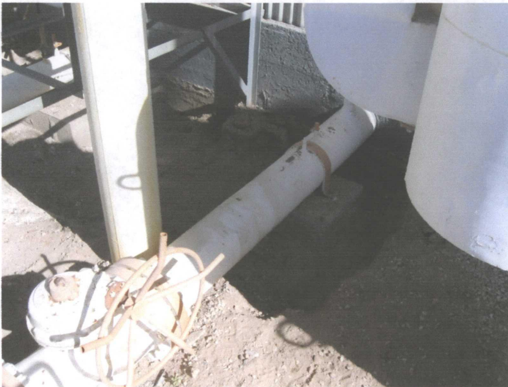
Photo 10 - Compressor area 13 excavation looking west/northwest
