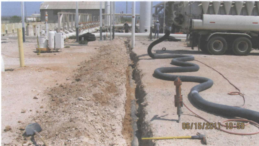
Photo 27 – Pipe #16 removal looking north toward Compressor Building and former Cooling Tower from termination of pipe.
