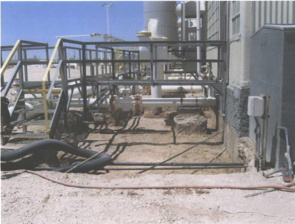
Photo 6 - Compressor area 9 excavation, looking west
