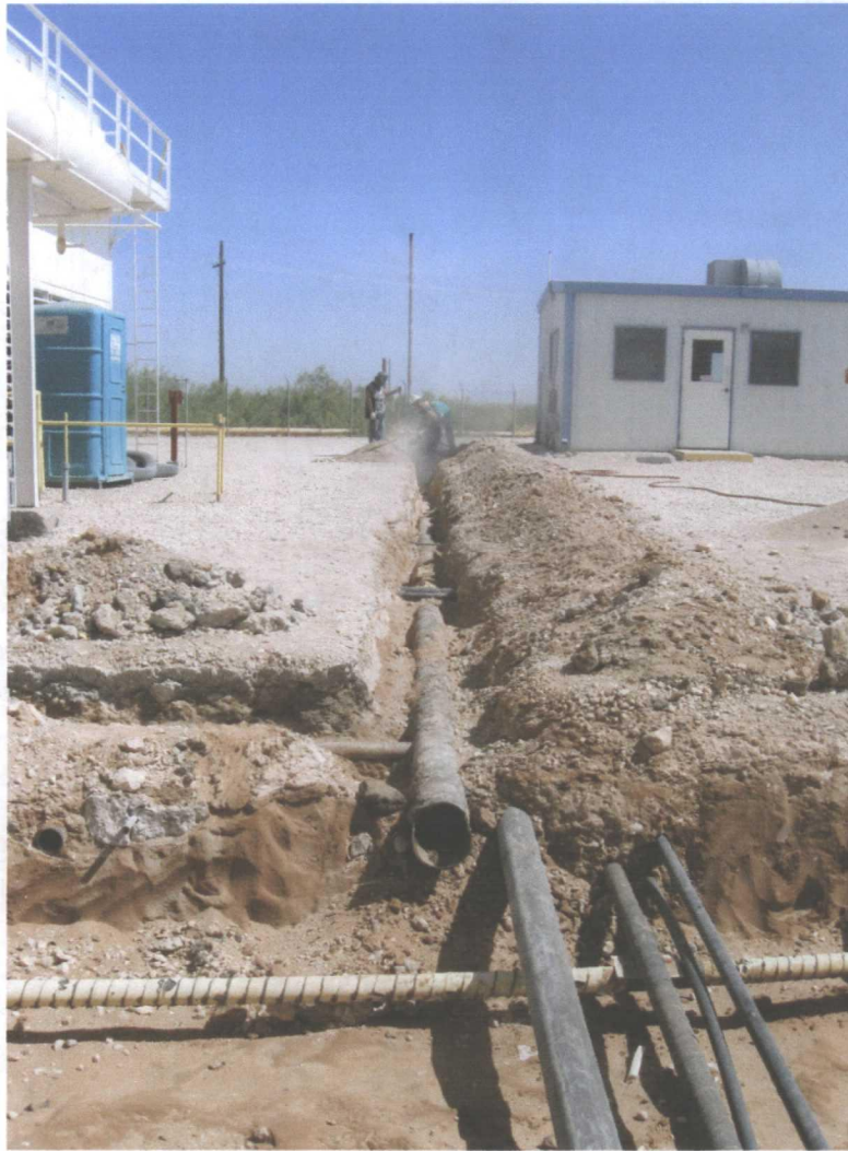
Photo 22 - Excavation of the Pipe #2 trench to remove piping traveling north. Note secondary pipe connecting to Pipe #2 in foreground.
