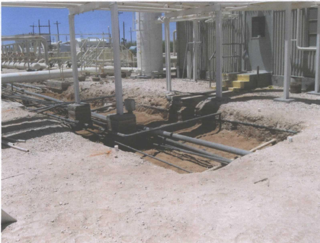
Photo 20 - West Compressor Building excavation on the north side
