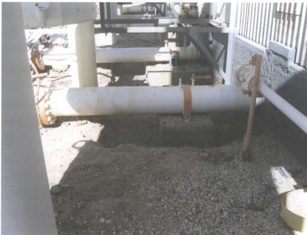
Photo 11 - Compressor area 13 Excavation looking west
