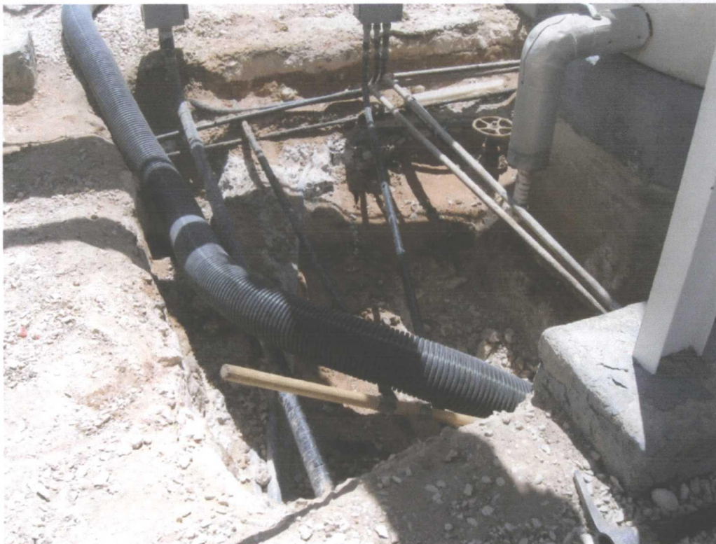
Photo 14 - Completed excavation at Jacket Water Tank
