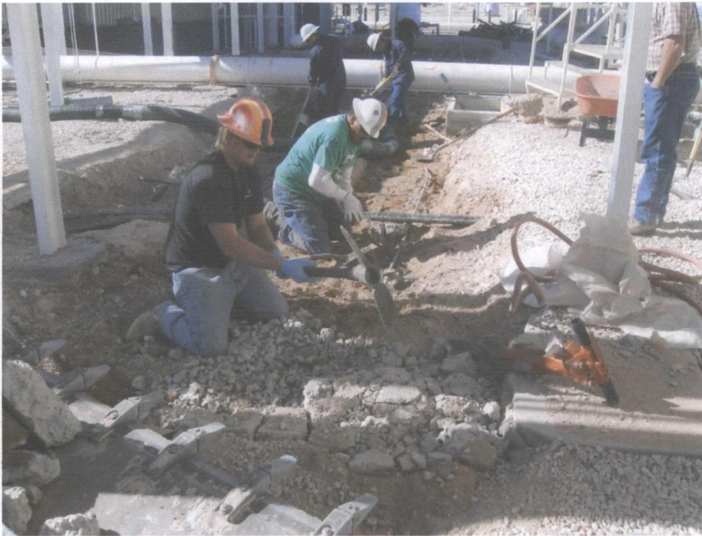
Photo 19 - On-going excavation at the West Compressor Building
