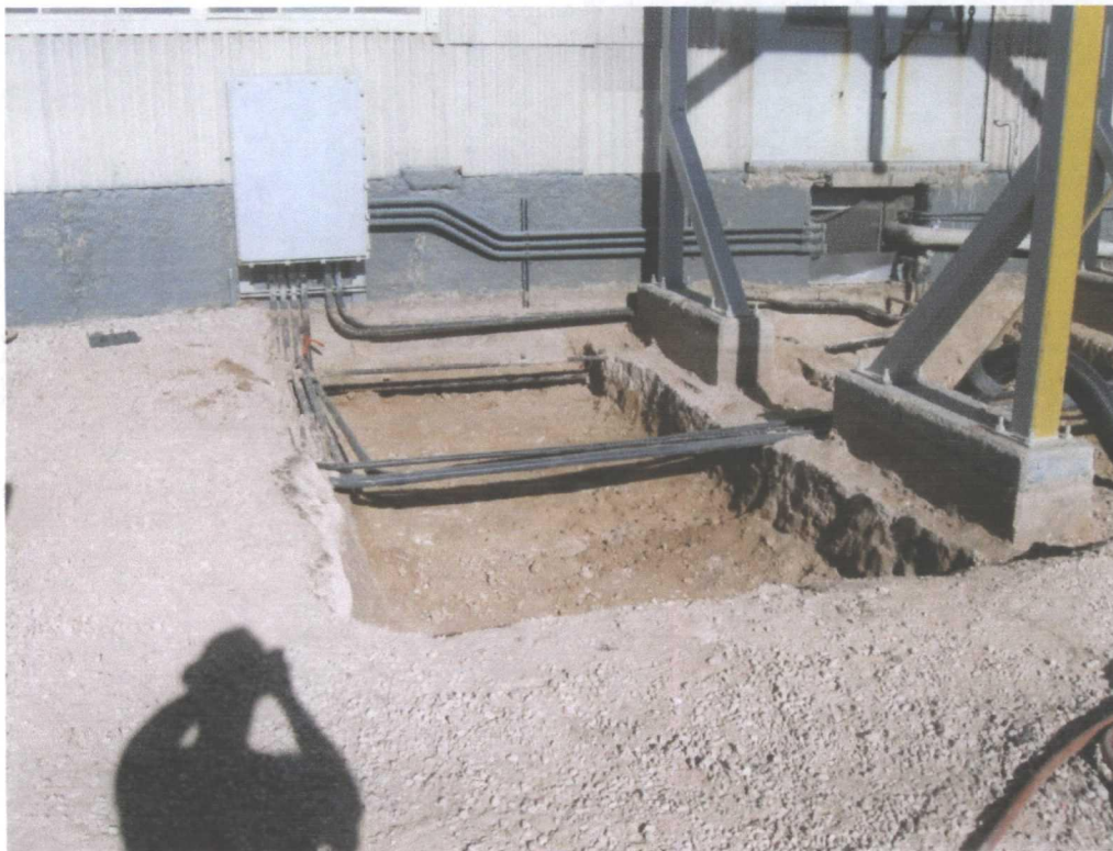
Photo 4 - Compressor area 8 excavation looking west at south half of excavation
