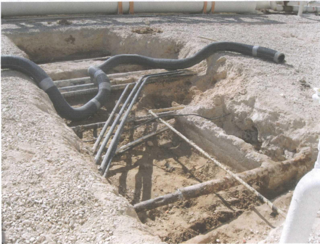
Photo 16 - Beginning of excavation at the West Compressor Building
