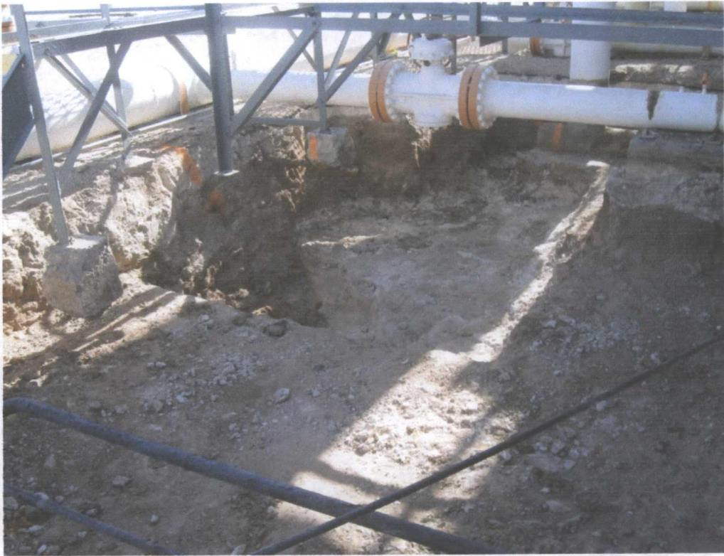
Photo 7 - Compressor area 9 excavation after removing additional soils
