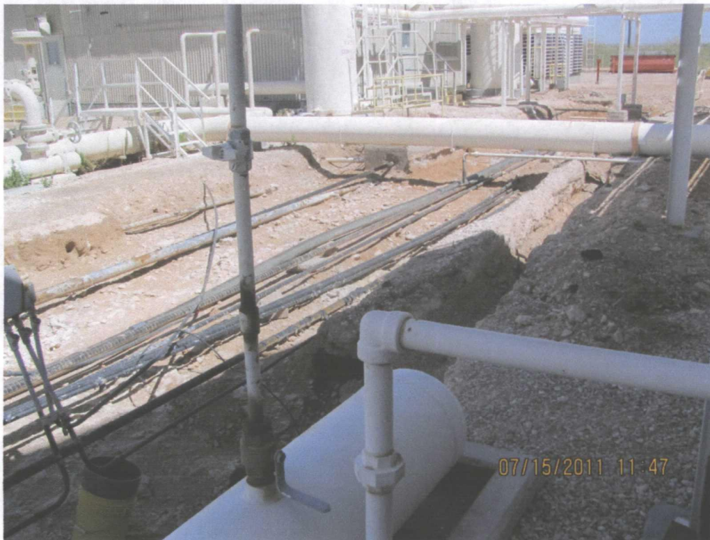
Photo 25 – Pipe #6 removal looking north from waste oil transfer tank. Pipe #6 was removed from trench adjacent to the main excavation.
