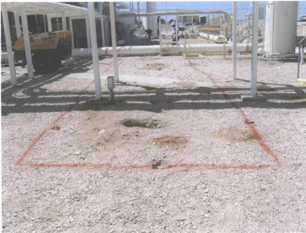
Photo 15 - Excavation area for West Compressor Building marked
