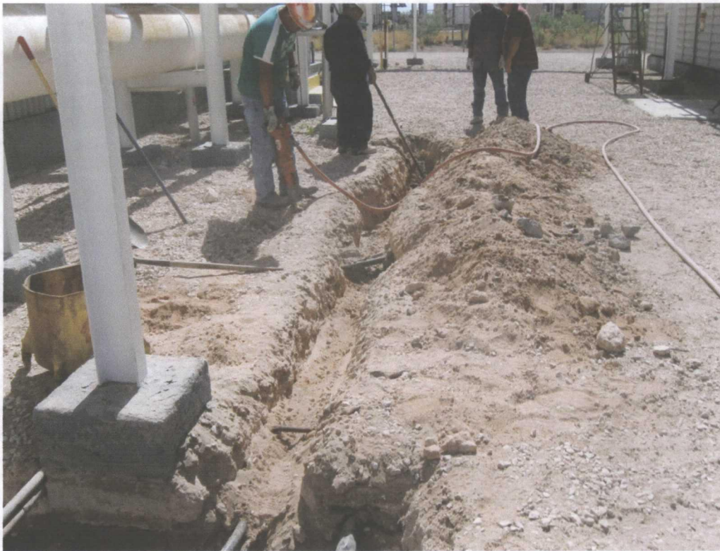
Photo 24 – Secondary pipe removal looking west between West Pump Room and Fin Fan, taken from Jacket Water Tank
