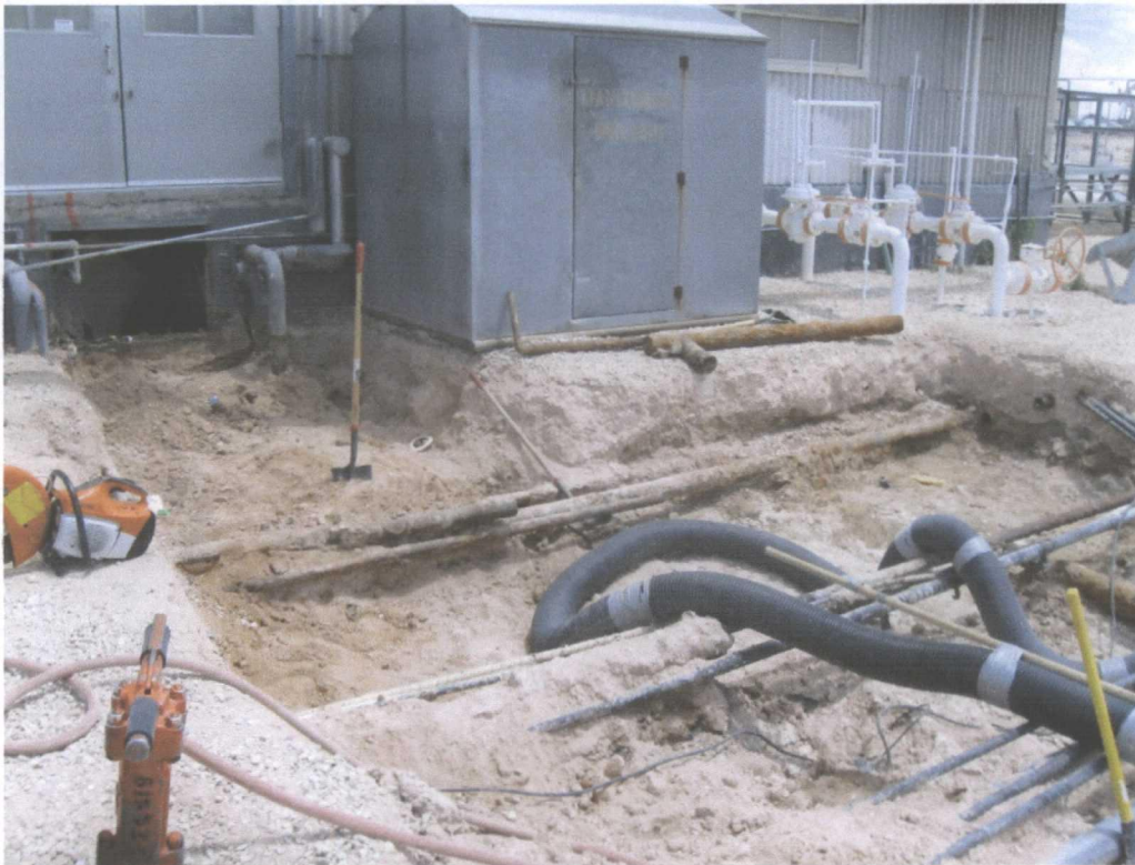
Photo 17 - On-going excavation at the West Compressor Building
