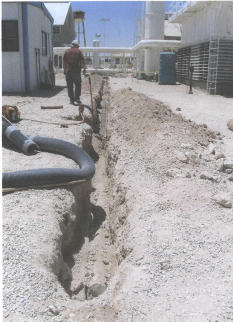
Photo 23 - End of the trench looking south for Pipe #2 removal
