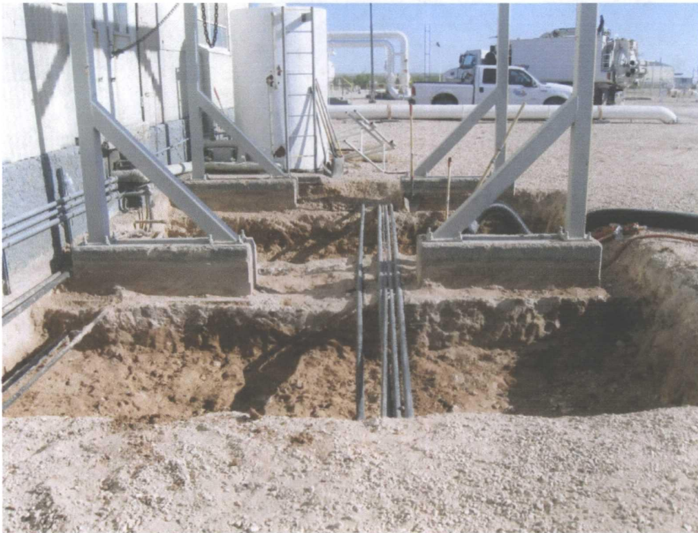
Photo 2 - Compressor area 8 excavation completion looking north
