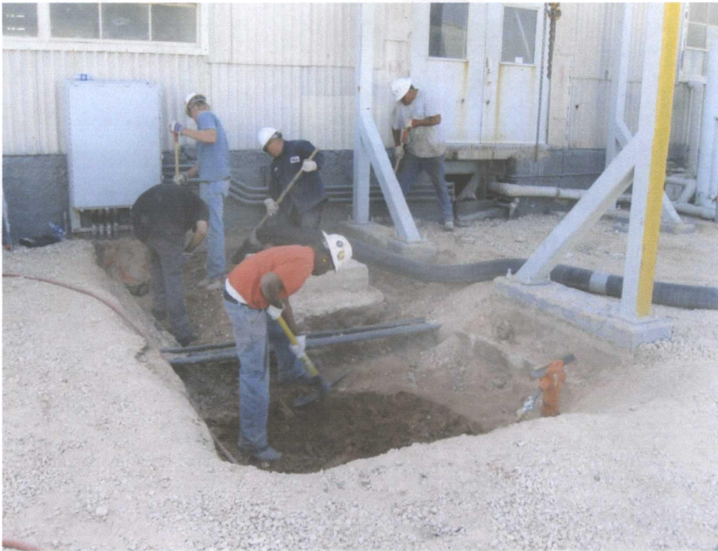
Photo 1 - Compressor area 8 excavation initiation looking west
