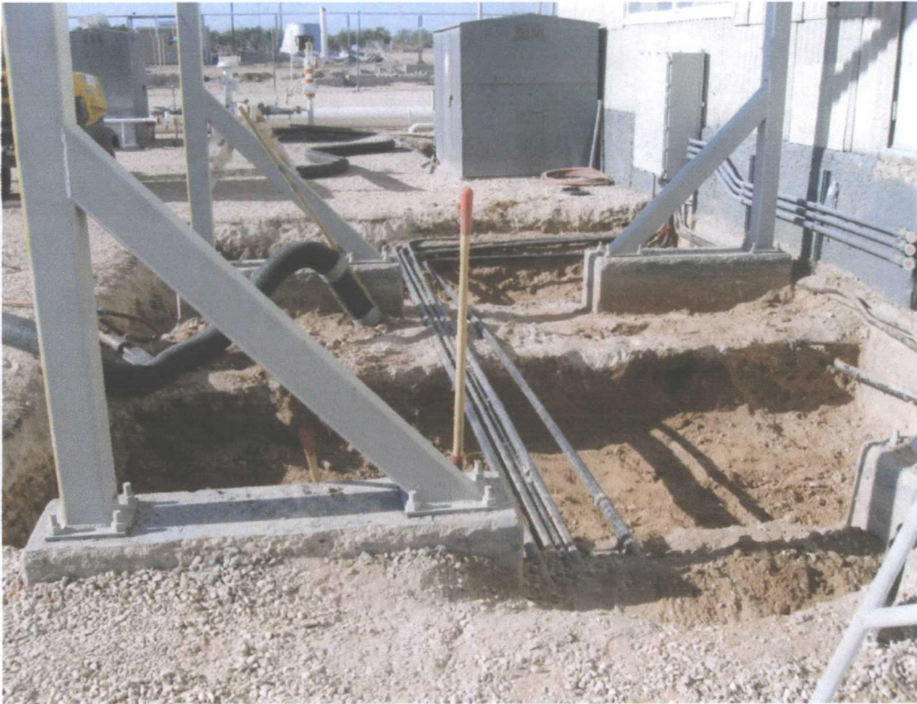
Photo 5 - Compressor area 8 excavation looking south
