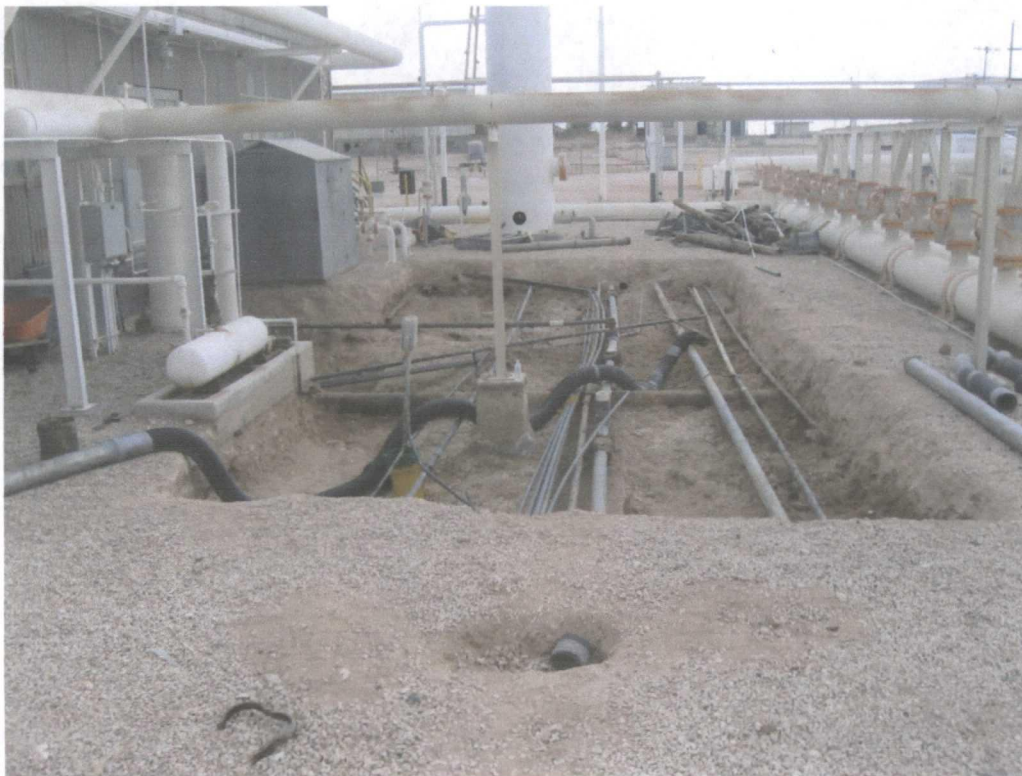
Photo 18 - On-going excavation at the West Compressor Building
