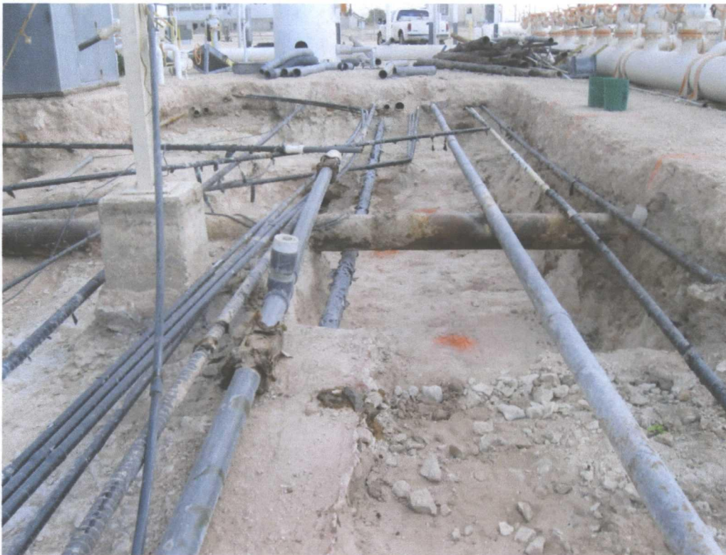
Photo 21- West Compressor Building additional excavation completed in the areas where concentrations were over the CULs
