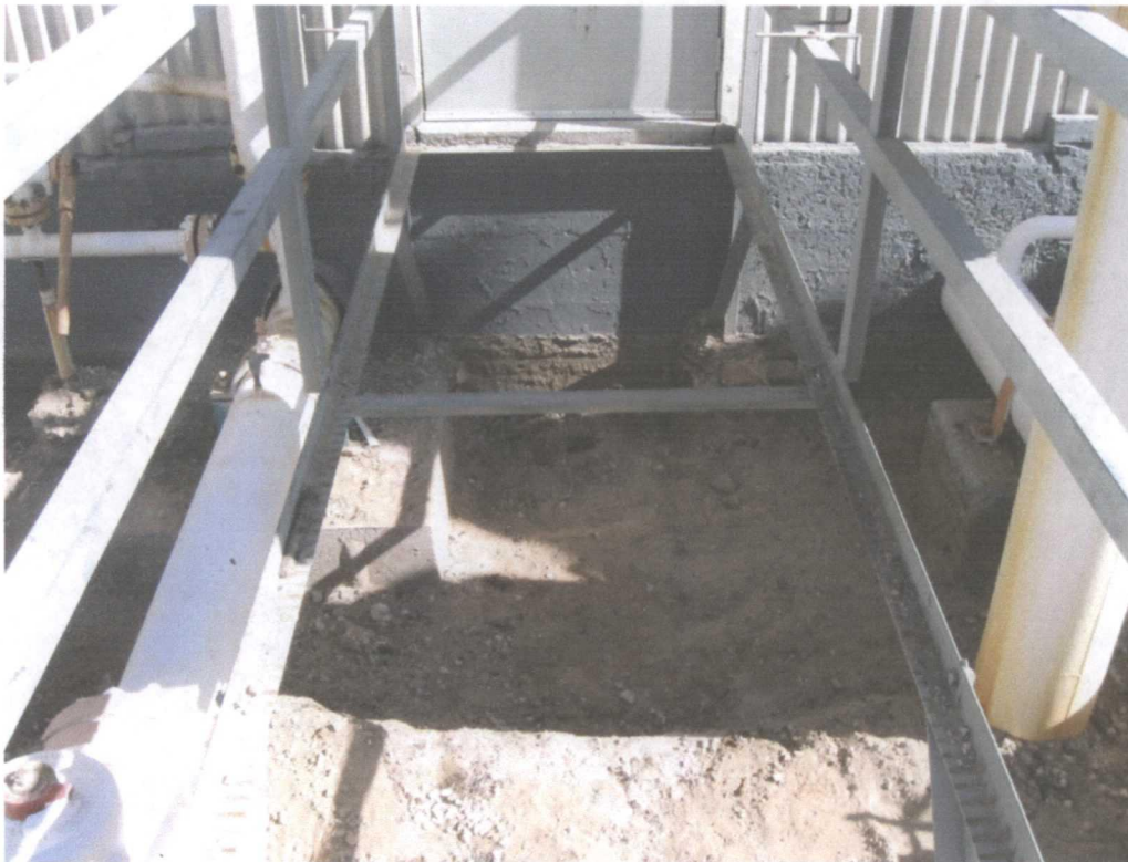
Photo 9 - Compressor area 13 excavation looking north
