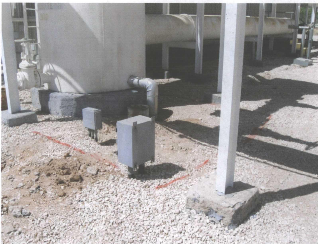
Photo 12 - Excavation area marked for Jacket Water Tank
