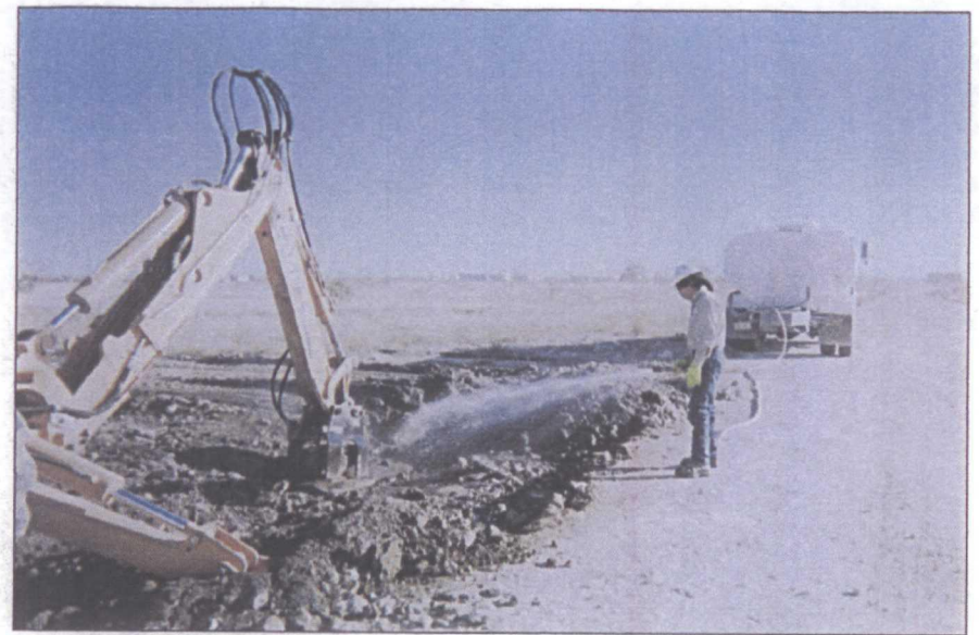
backfilling and compacting
