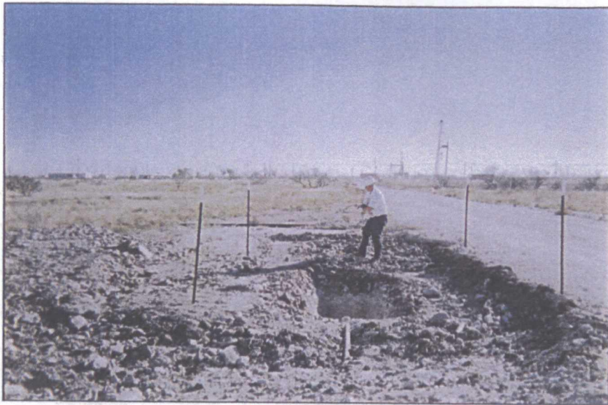
delineation trench before backfilling
