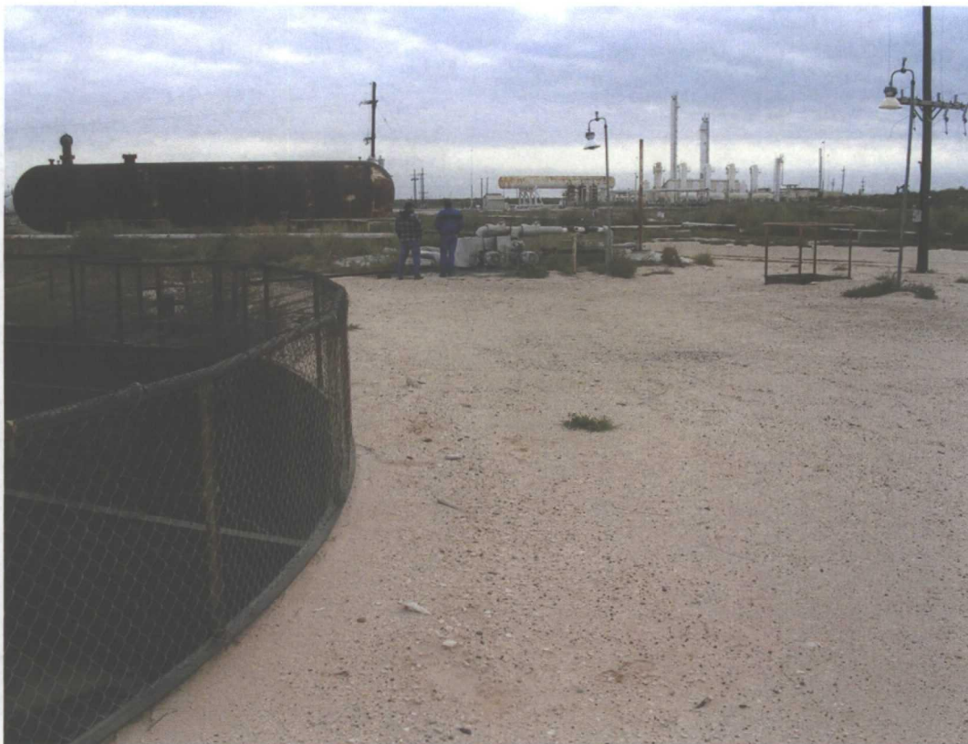
Surge Tank (Left) and Below Grade Classifier and Waste Oil Storage Tanks
