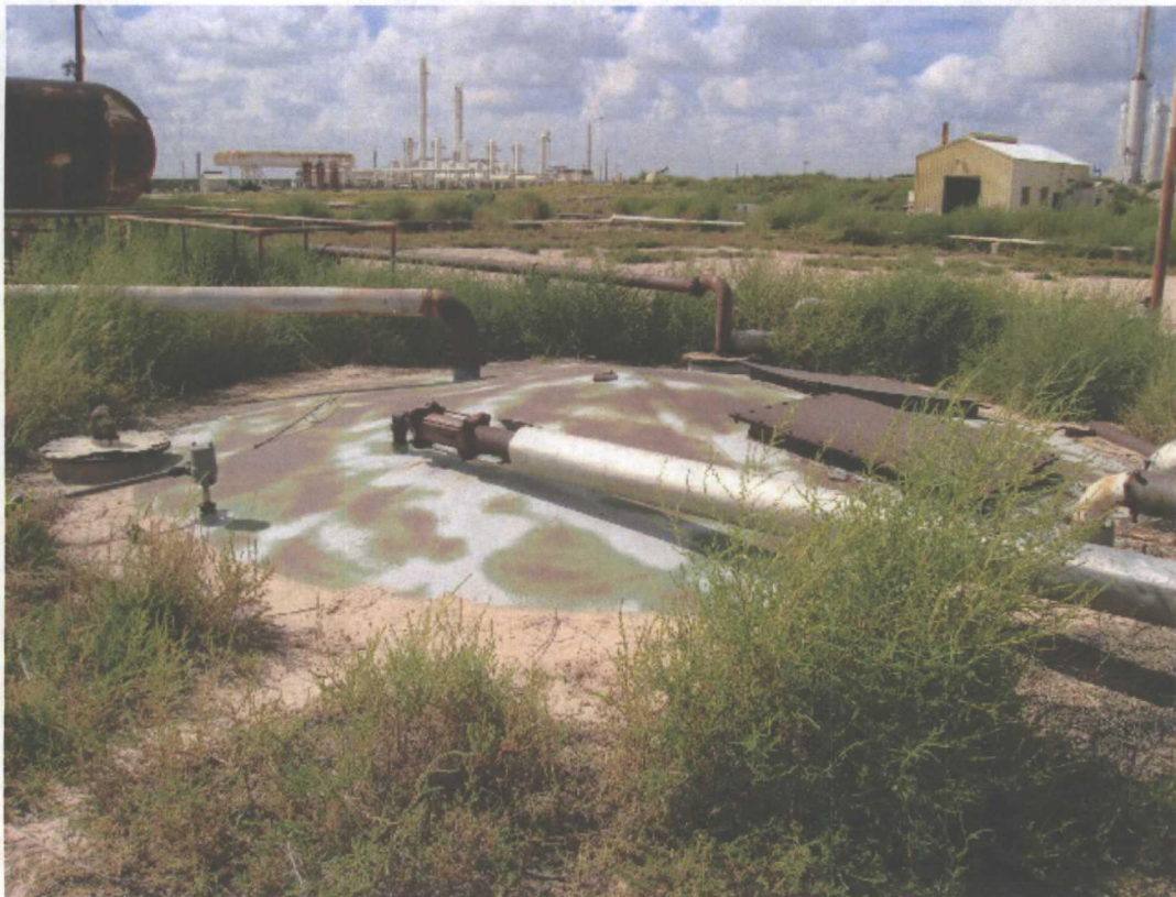
Close Up of Below Grade Classifier
