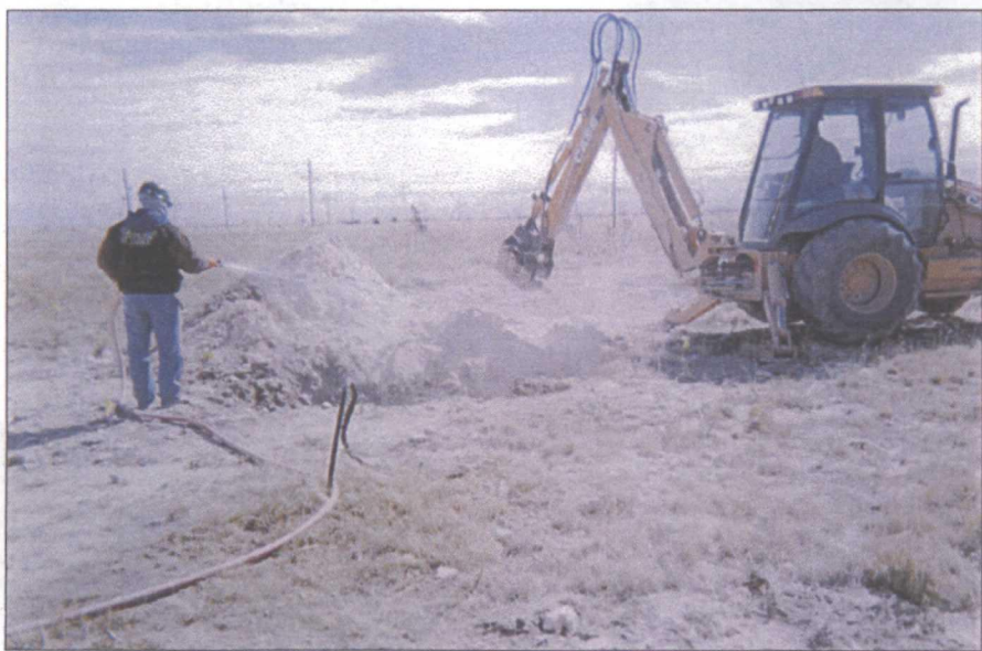
backfilling delineation trench
