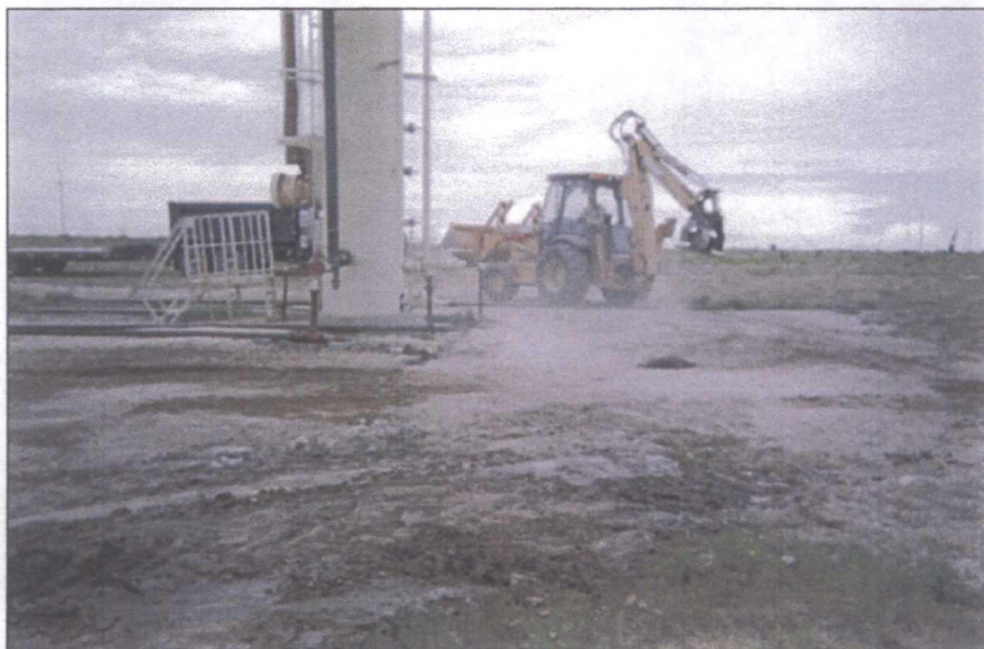
backfilling
