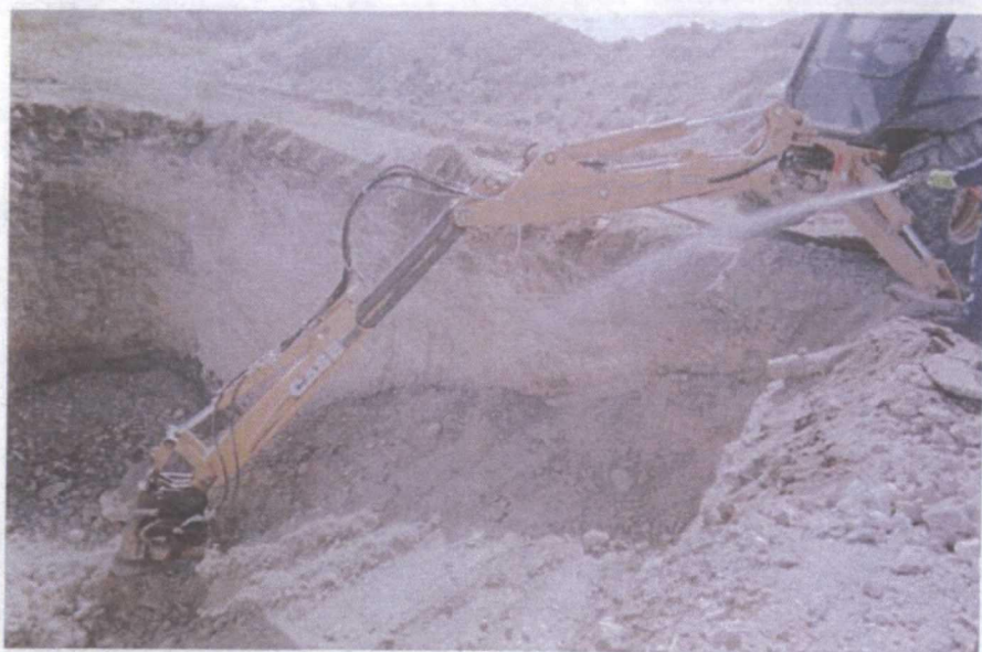
backfilling excavation site, facing north
