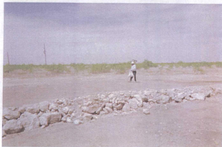
seeding backfilled site
