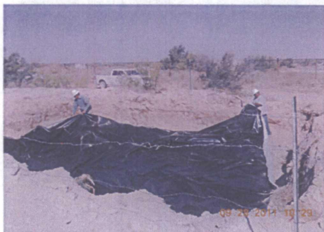
Installing liner, facing northwest
