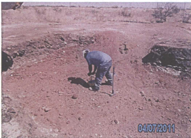
Compaction test on clay liner, facing north 4.7.11
