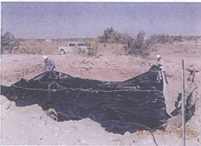
Installing liner, facing northwest 9.28.11
