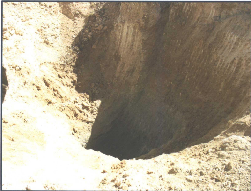
Photograph #8: Additional view of excavation area S-1, excavator teeth having difficulty breaking up caliche
