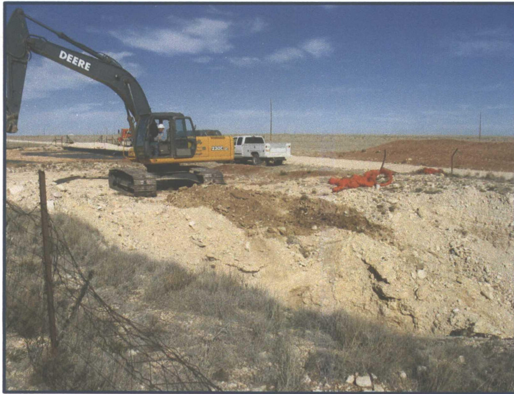
Photograph #5: View of excavator preparing site in order to access the southeast and previously most contaminated portion of the existing pit.
