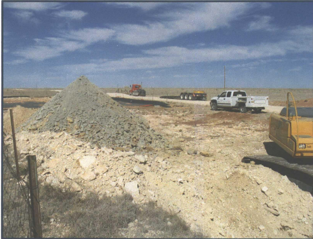
Photograph #9: Greyish material excavated from S-1, initially thought to possibly be grout from abandoned well but determined to be stained caliche as field PID readings indicated petroleum contamination.
