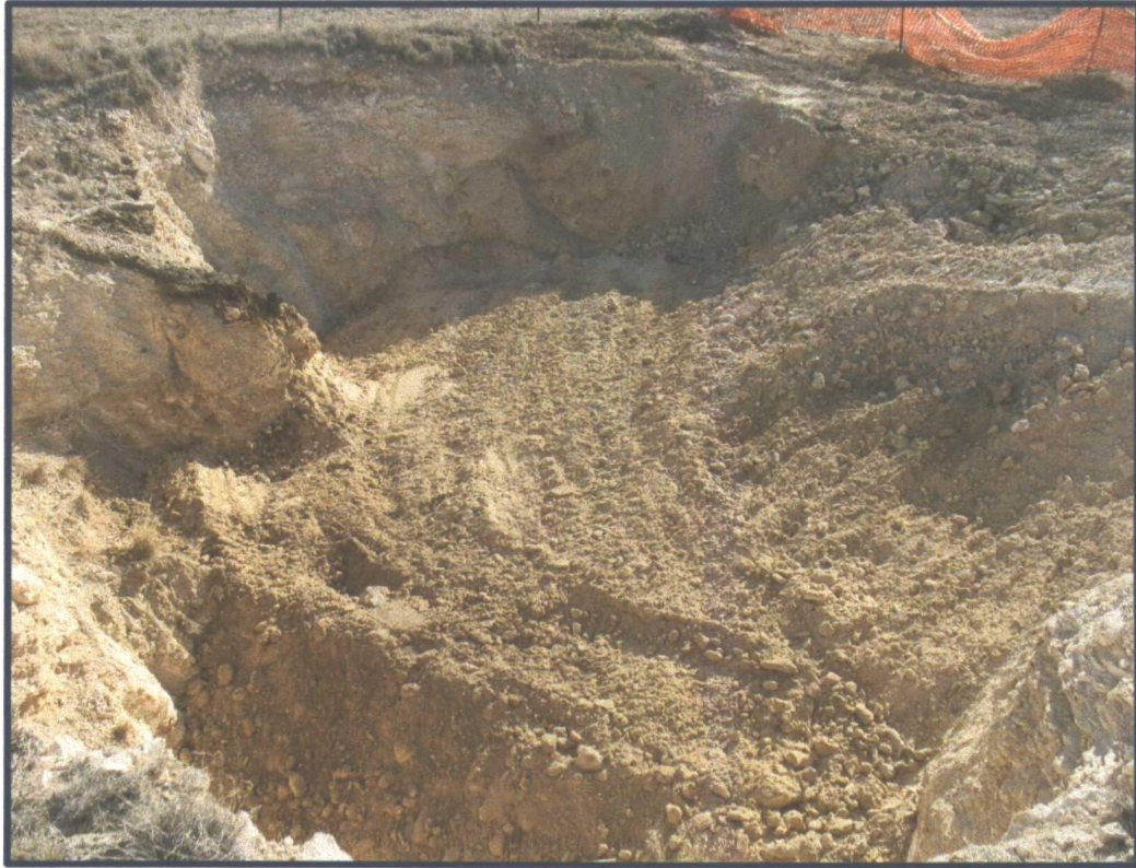
Photograph #19: Benching and ramp construction of existing pit for added site safety and ingress/egress of any livestock that may get beyond the current fencing around the pit.
