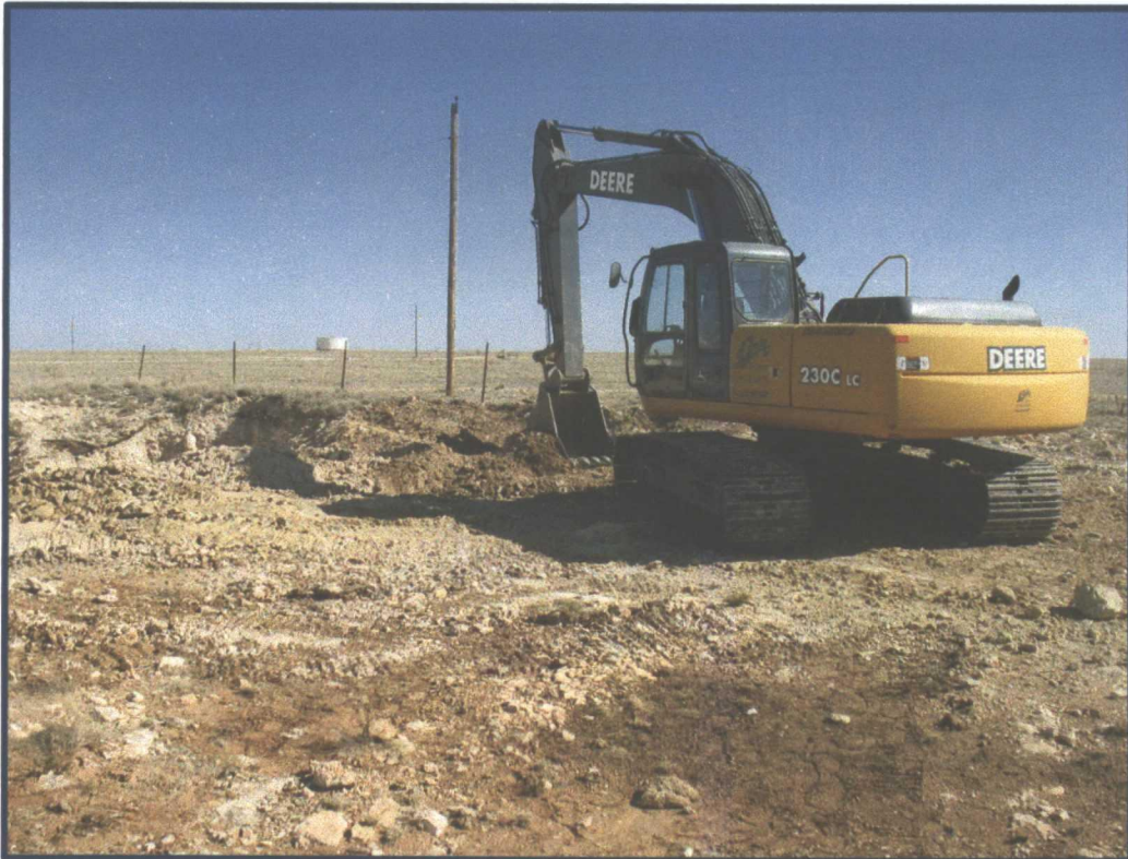
Photograph #18: Excavator backfilling pot-hole area S-4.
