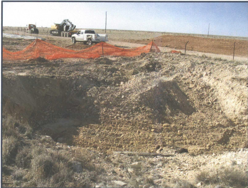
Photograph #20: Additional view of large pit benched, ramped and with netting added for additional visibility/safety.
