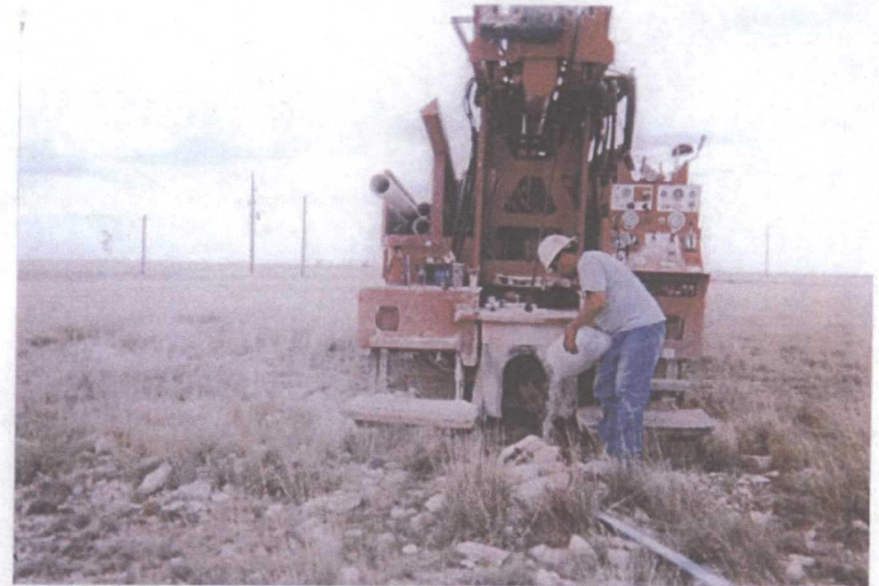
plugging SB #1 with bentonite
