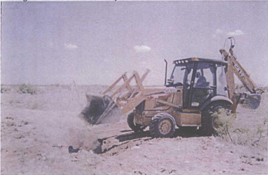
backfilling the former junction box site, facing northwest
