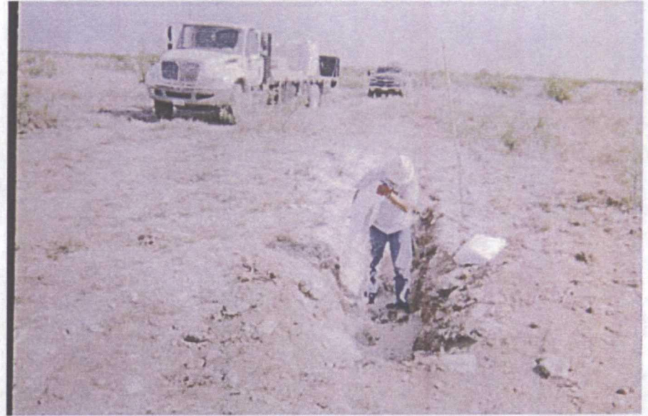
plugging SB #1 with bentonite
