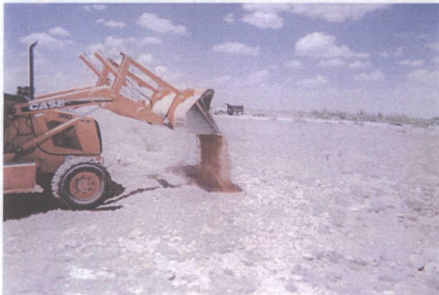
backfilling the former junction box site with clean soil
