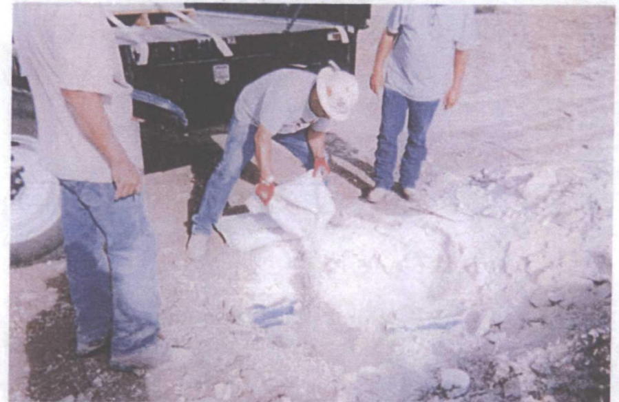
plugging SB #1 with bentonite
