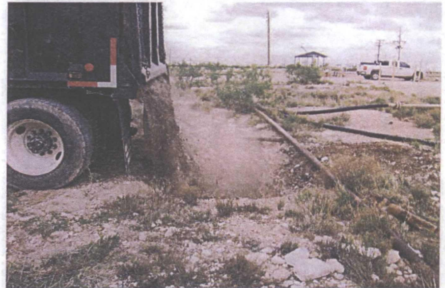
backfilling the excavation
