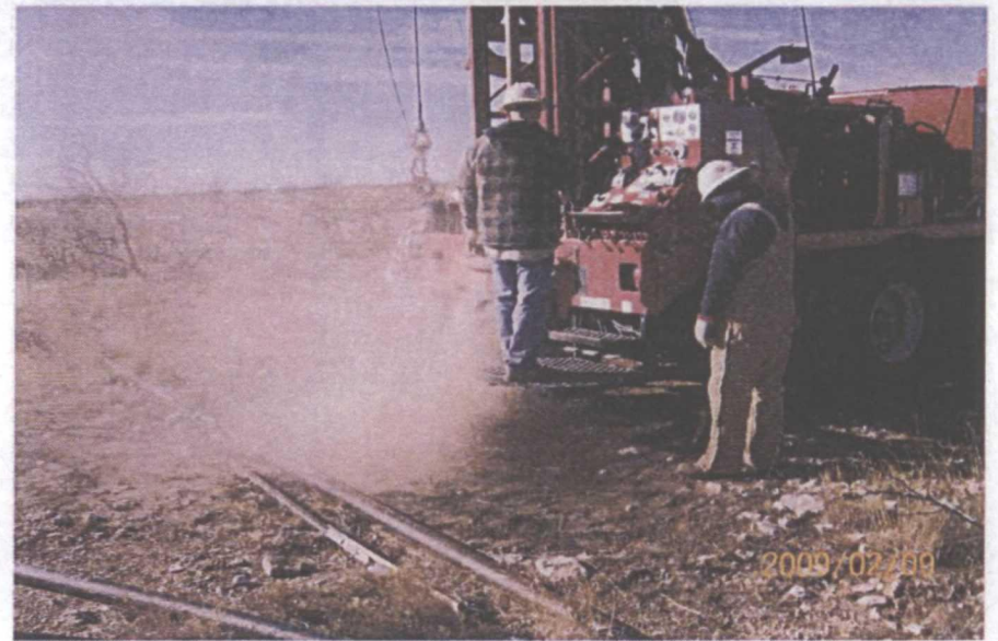
soil boring the former junction box site
