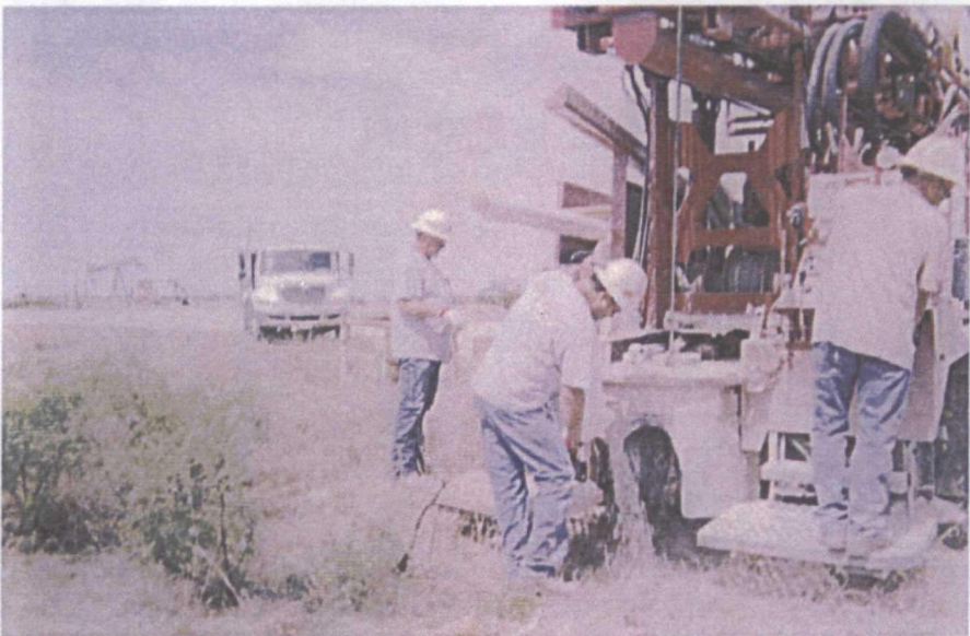
plugged SB #1 with bentonite
