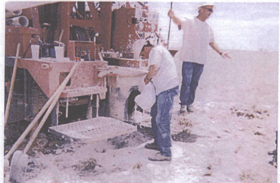
plugging SB #1 with bentonite
