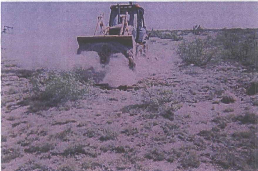
Backfilling excavation
