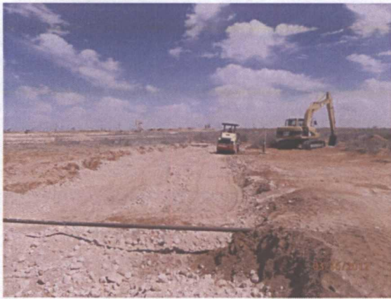
Roller packing caliche in backfilled excavation, facing east 3/16/12
