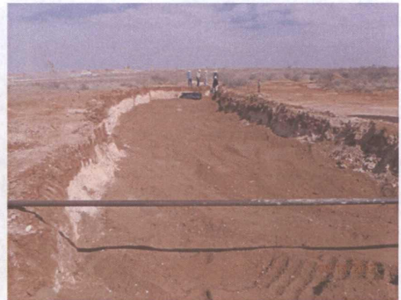
Installed bottom 6" sand pad, facing east 3/15/12
