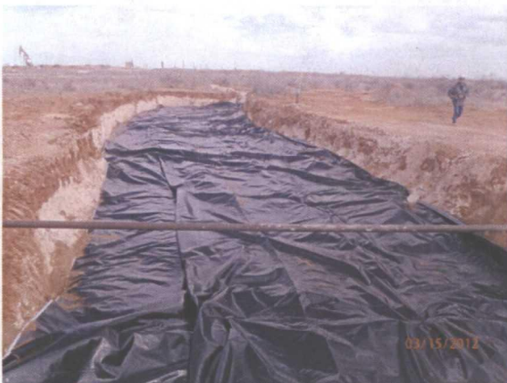
Installed 115' x 25', 20-mil reinforced plastic liner, facing east 3/15/12
