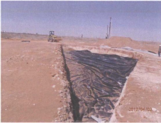
Installed north portion of 20-mil reinforced plastic liner, facing east 4/2/12
