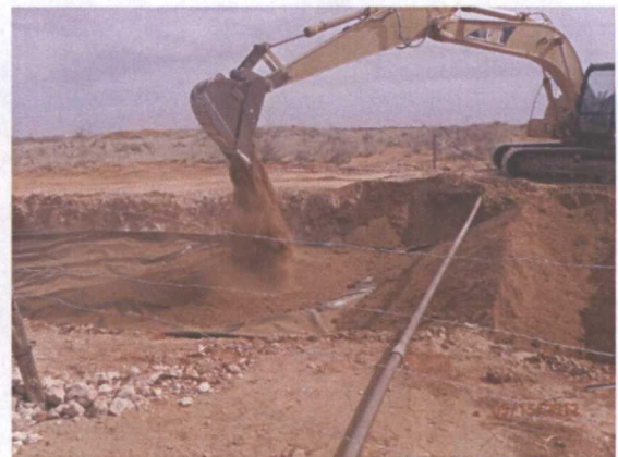
Installing 6" sand pad above liner, facing east 3/15/12
