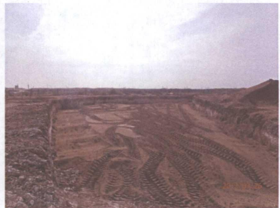
Installed bottom 6" sand pad, facing east 3/26/12
