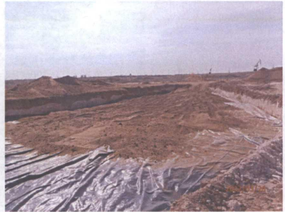
Installing 6" sand pad above liner, facing west 3/26/12
