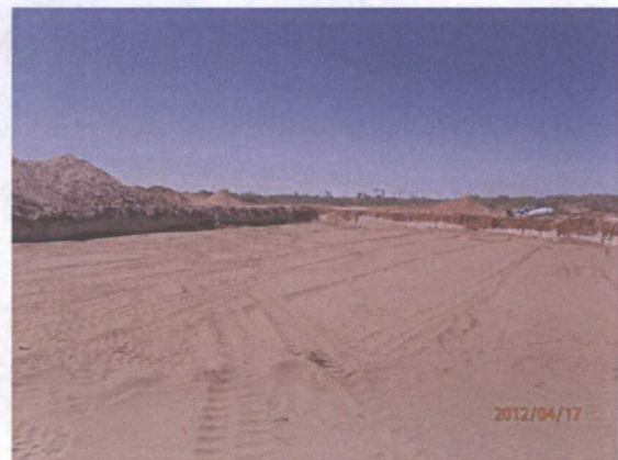
Installed bottom 6" sand pad, facing southwest 4/17/12
