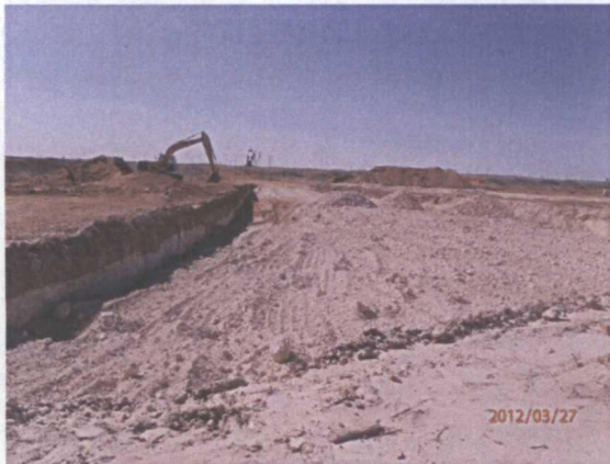
Backfilling site with caliche, facing west 3/27/12
