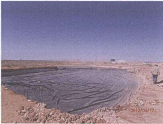
Installed 190' x 130', 20-mil reinforced L-shaped plastic liner, facing northeast 4/17/12
