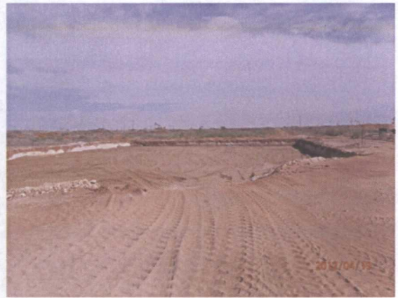
Installed 6" sand pad above liner, facing north 4/19/12
