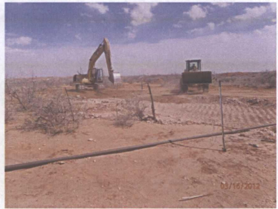
Backfilling 2' deep excavation with sand to ground surface, facing southeast 3/16/12
