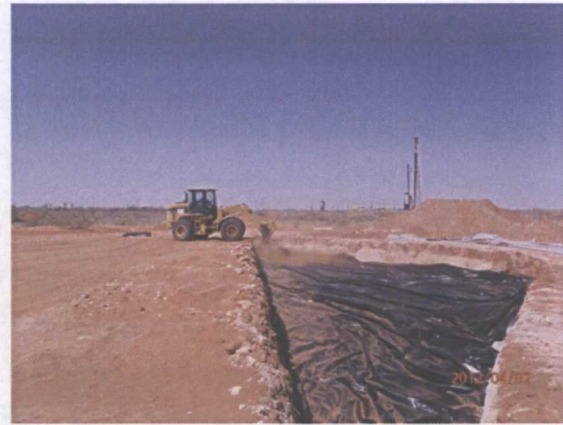
Backfilling excavation with imported sand, facing west 4/2/12
