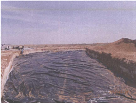
Installed south portion of 85' x 180', 20-mil reinforced plastic liner, facing east 3/26/12
