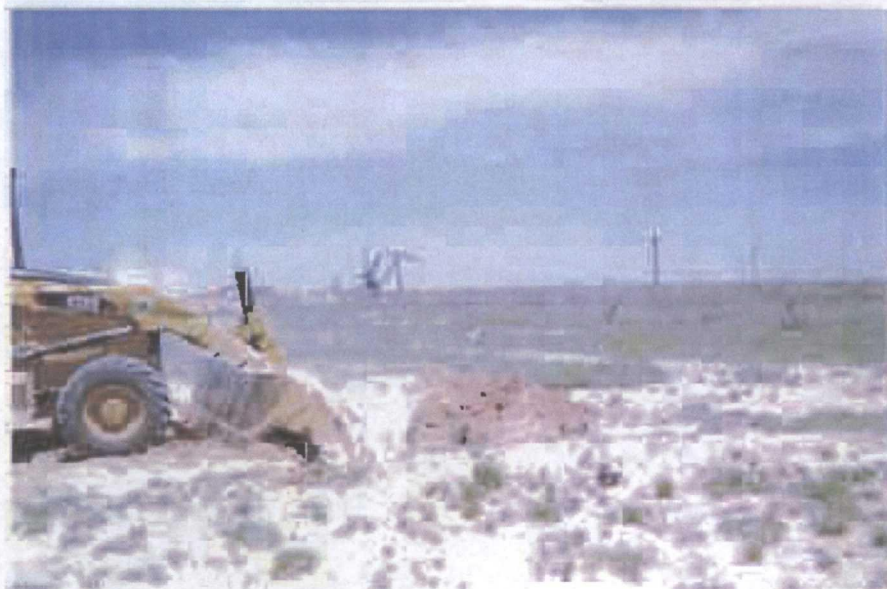
Backfilling excavation
