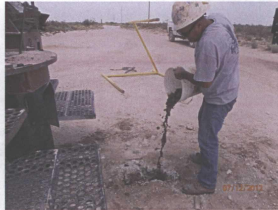
Pouring the 1-3% bentonite/concrete slurry into bore hole, facing north
