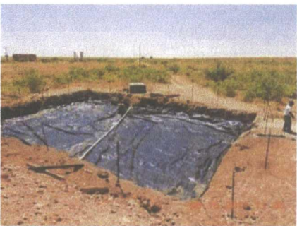
20-mil reinforced liner installed, facing southeast 8.15.11
