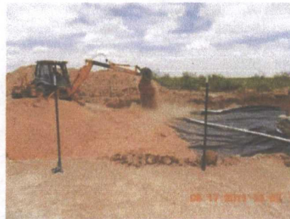
importing sand for 6" pad above liner, facing west 8.17.11
