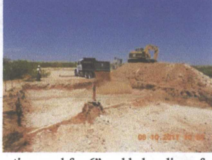
importing sand for 6" pad below liner, facing northwest 8.10.11
