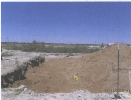
Installed 1' sand pad above liner, facing west 7/31/2012
