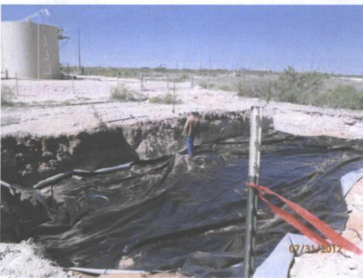
Installed 18' x 52', 20-mil reinforced plastic liner, facing southwest 7/31/2012
