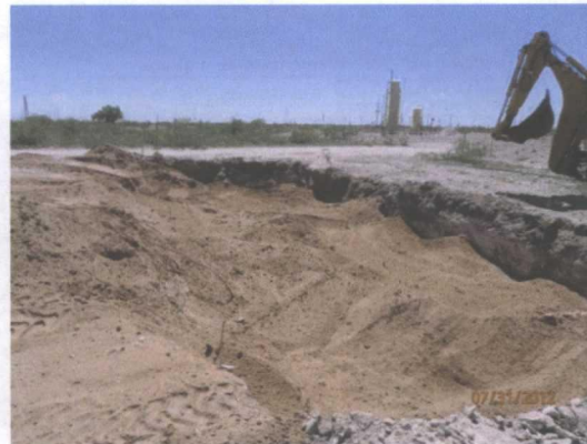
1' sand pad above liner, facing east 7/31/2012
