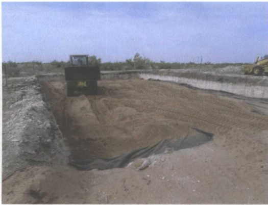
Installing 1' sand lift above liner, facing south 8/17/2012
