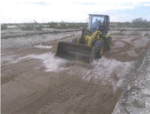
Installing 6" bottom sand pad, facing south 8/15/2012
