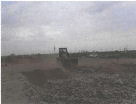
Backfilling with topsoil from 2' bgs, facing north 8/17/2012
