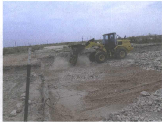
Returning rock to 2' bgs, facing east 8/17/2012
