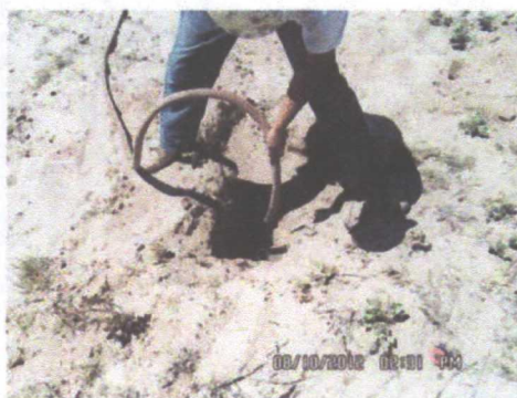
Each MW was filled with Cement Type I-II and 1-3% bentonite grout.
