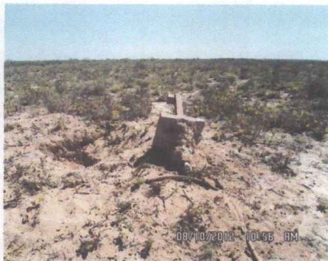
Typical removal process- dug around MW and hand cut pipe and removed with rig.
