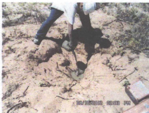
Topping of each hole to counter slumping.
