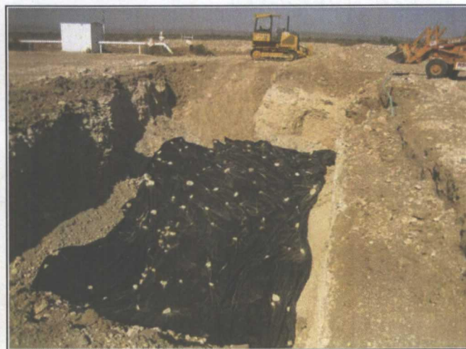
6.) View of plastic liner within on-site excavation prior to backfill activities, looking west.
