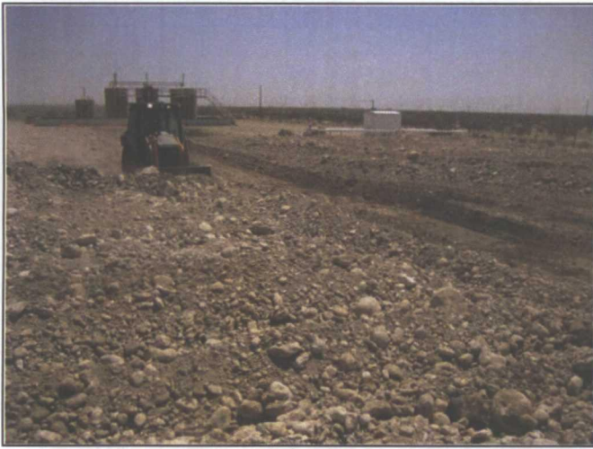
7.) View of treated soils used for partial excavation backfill, approximately 100 cubic yards total, looking east.
