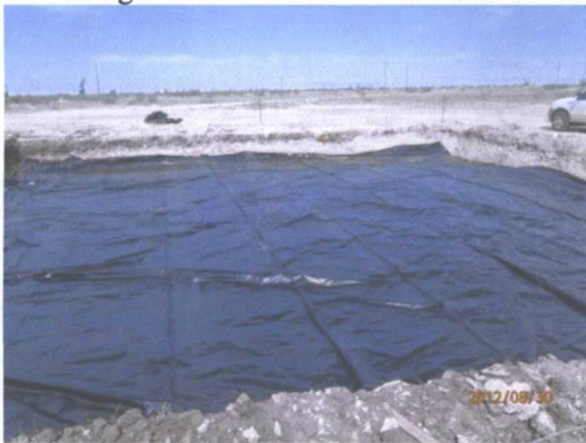
20-mil, reinforced liner installed, facing west 8/30/2012
