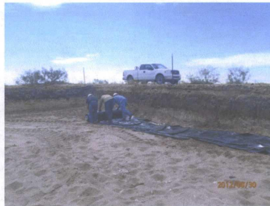
installing the 20-mil, reinforced liner above the 6 inch blow sand pad, facing north 8/30/2012
