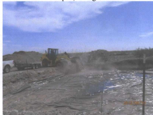
padding above the liner with 6 inches of blow sand, facing west 8/30/2012
