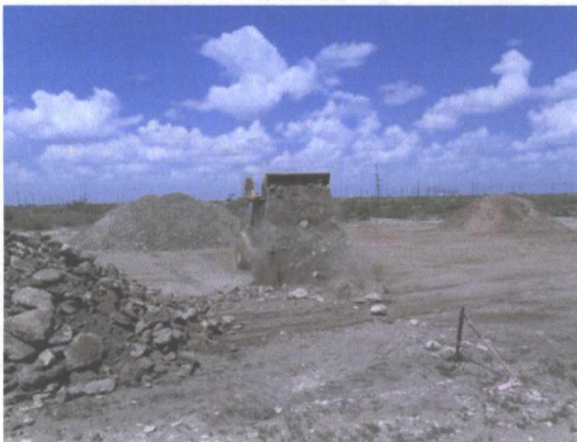
screening rock from the excavated soil, facing north 8/27/2012
