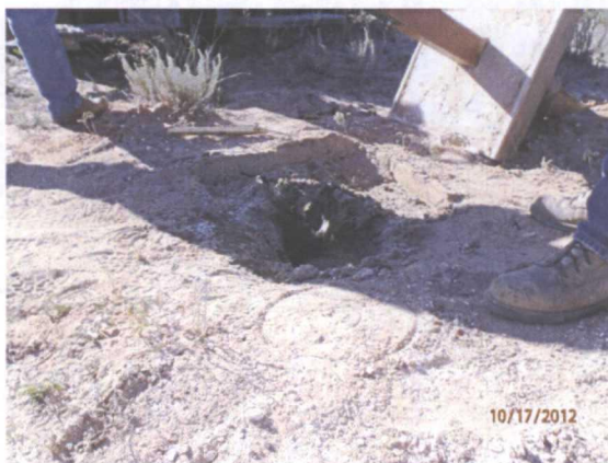
Plugging MW-3 with a 1-3% bentonite/concrete slurry with a 3 ft concrete cap 10/17/12
