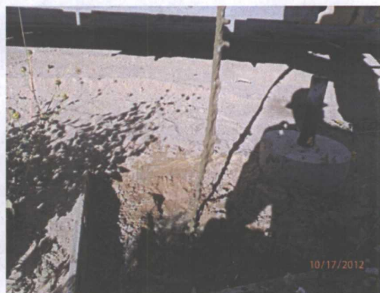
Plugging MW-1 with a 1-3% bentonite/concrete slurry with a 3 ft concrete cap 10/17/12
