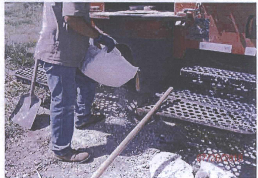
Soil Bore plugged with bentonite
