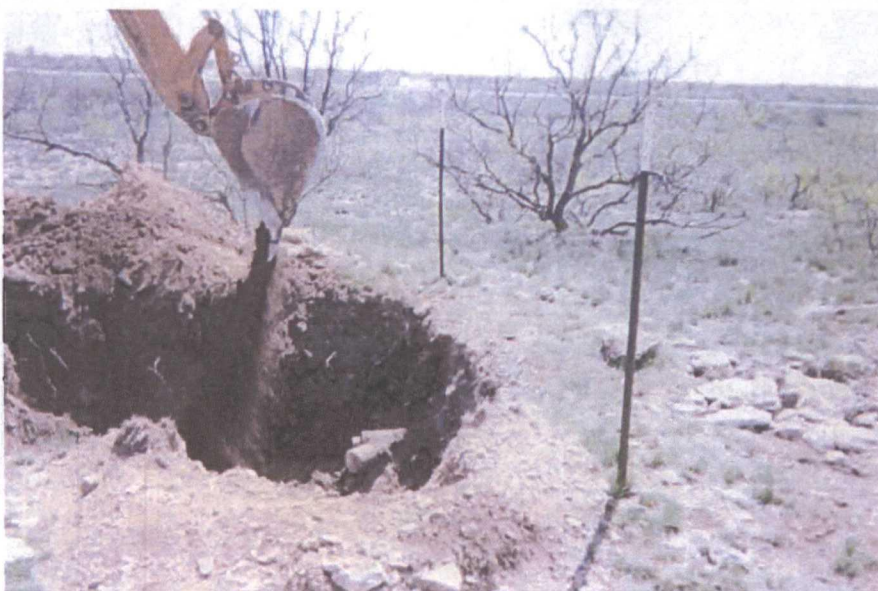
Backfilling excavation
