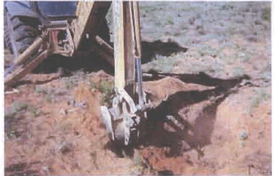
Delineation trench being excavated
