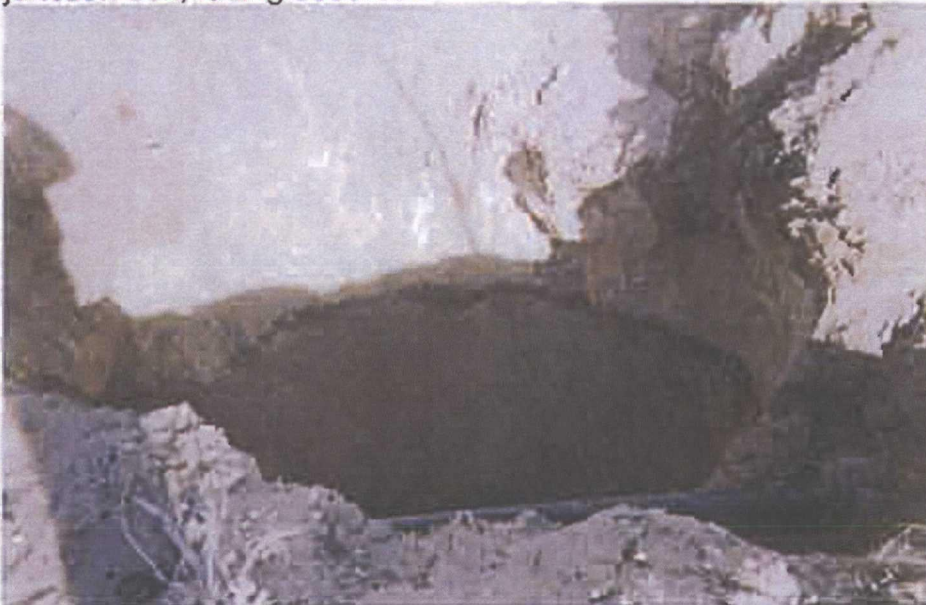
final 5x3x12-ft-deep excavation, facing north
