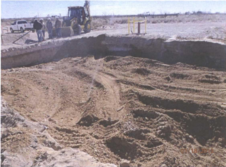
Installed a 3' pad of blow sand, facing southwest
