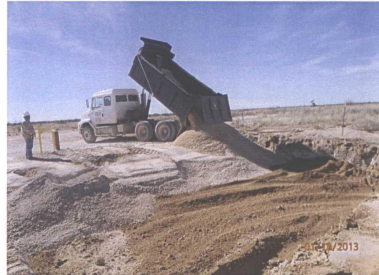
Importing caliche for backfill, facing southwest
