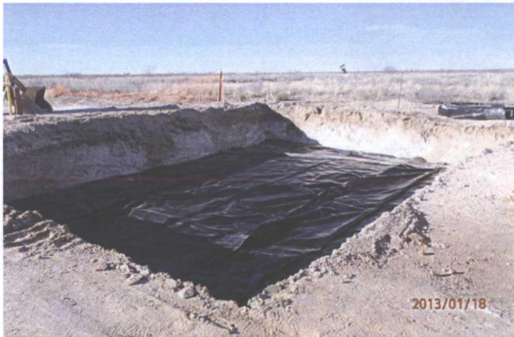
Installing liner @ 5' bgs, facing southwest
