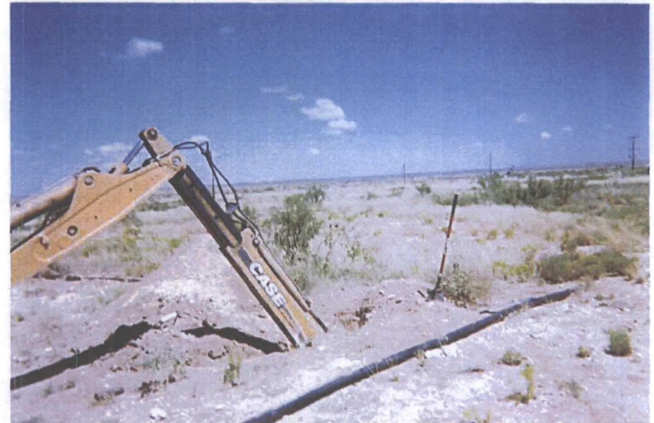
Delineation Trench being excavated
