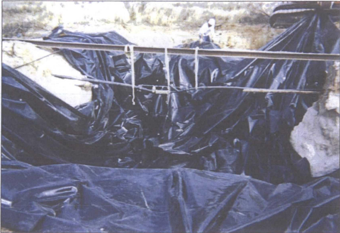
Installation of 20 mil Poly Liner
