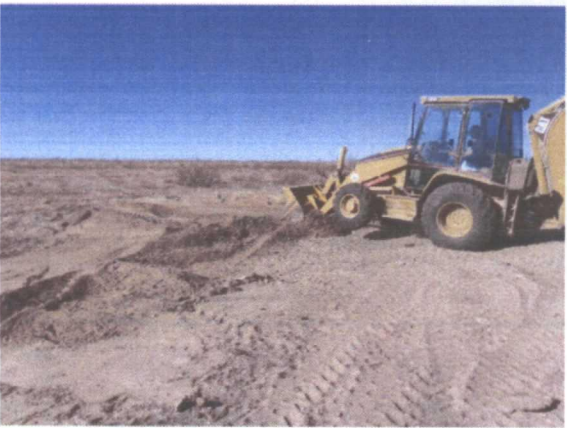
Backfilling the scraped area with clean, imported topsoil, facing west 12/12/2012
