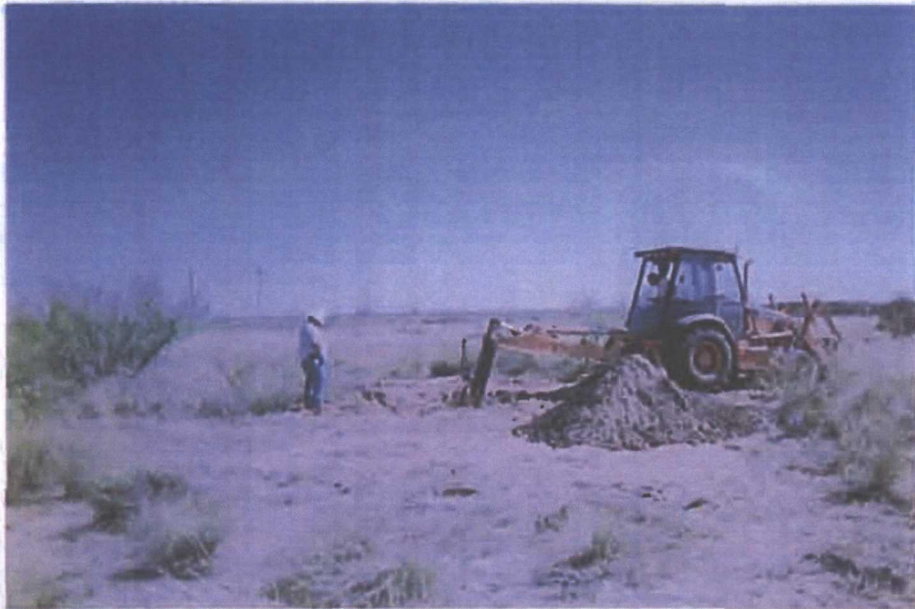
Delineation trench being excavated
