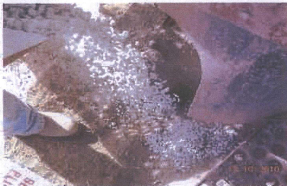
Plugging bore hole with bentonite
