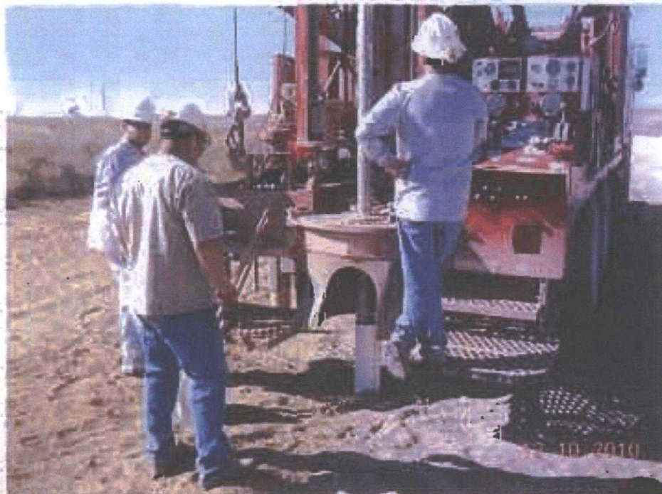
Drilling the soil bore
