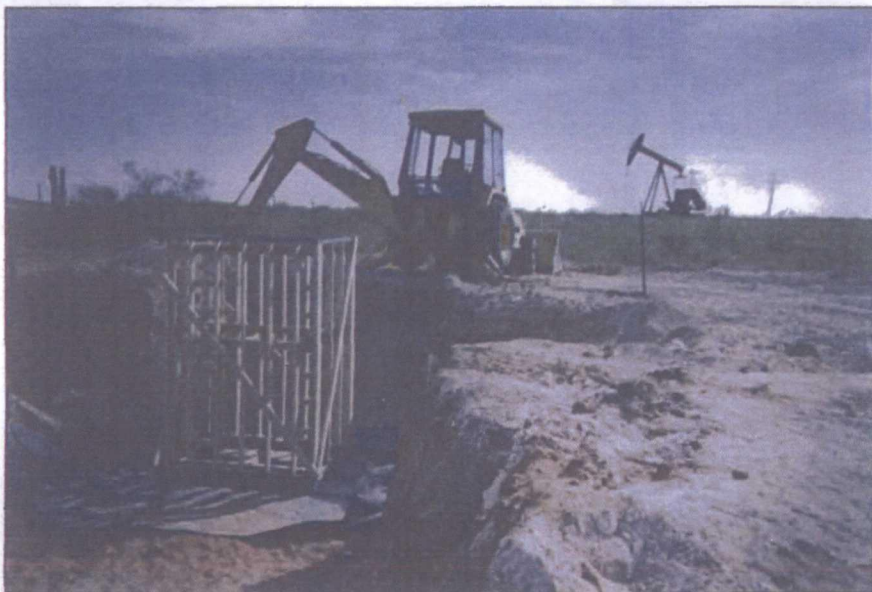
Construction of New Junction Box
