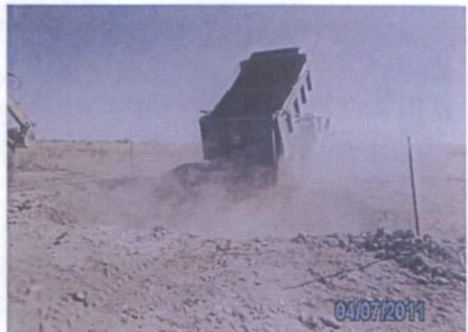
Backfilling site up to 5 ft BGS, facing northeast 4.7.11
