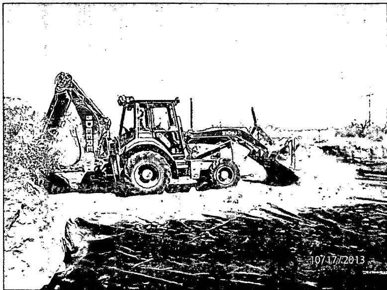
Backfilling over liner, facing east
