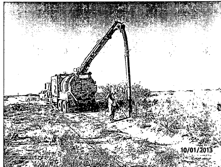
Line spot using hydrovac, facing north
