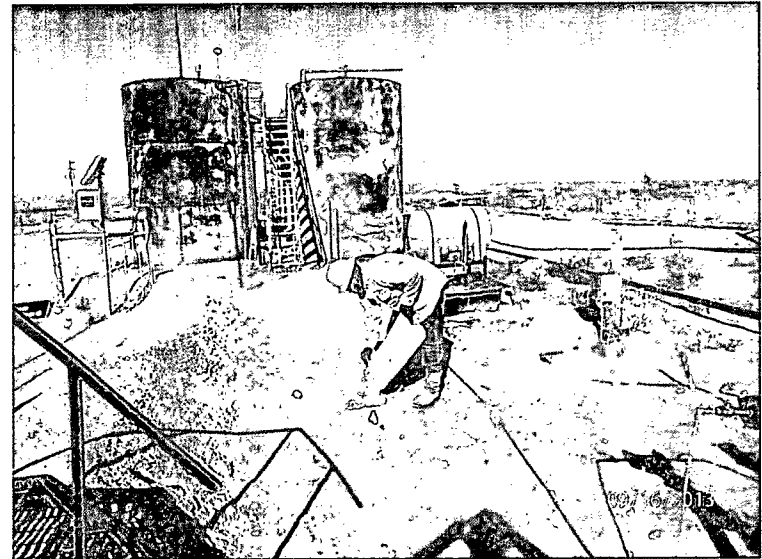
Plugging augur point in total with bentonite, facing west 9/16/13
