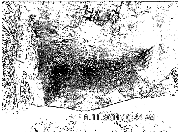
Clay layer in SB-1 excavation
