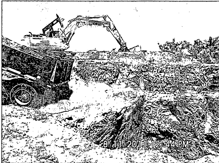
Importing sand to pad liners, facing north 8/11/11
