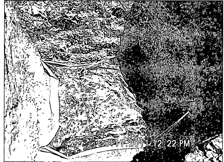
Installing poly liner in SB-1 excavation
