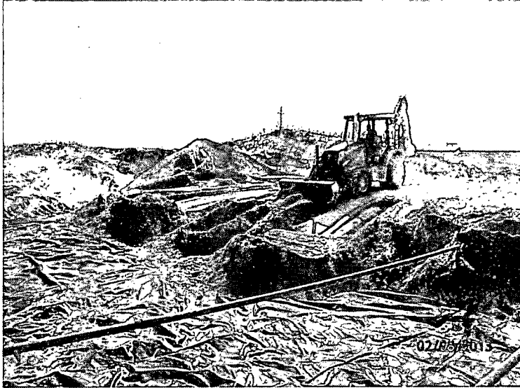
Backfilling above liner, facing east
