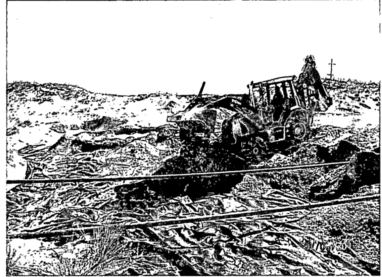
Backfilling above liner, facing east
