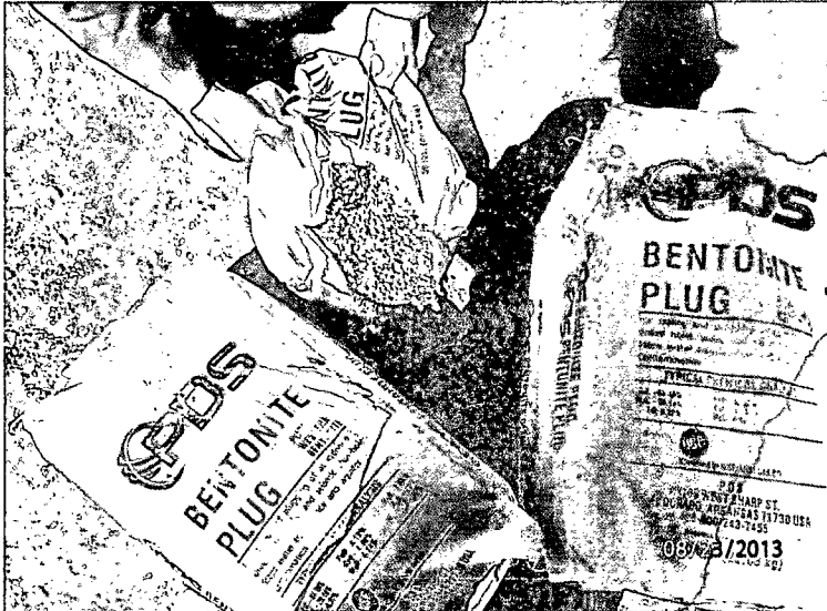
Plugging soil bore in total with bentonite
