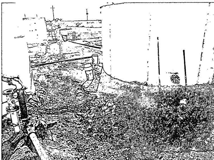
Backfilling Pt. 4 with clay, facing east
