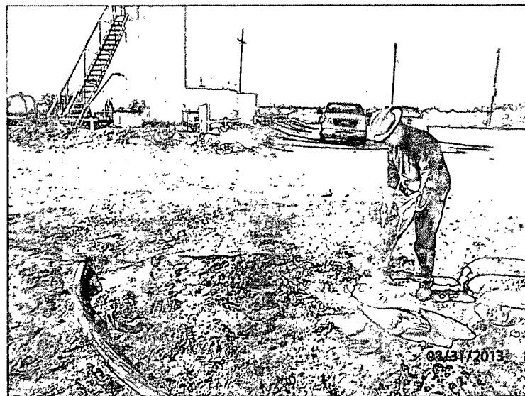
Plugging SB-2 in total with bentonite, facing south
