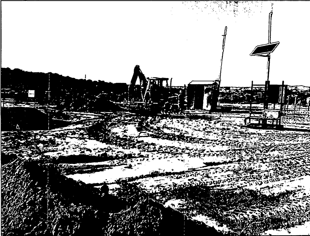
Photo 6: View of the Atlantic C #1A Meter Run backfill activities with imported soils.
