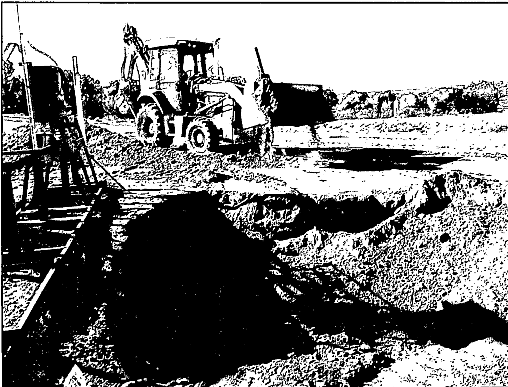
Photo 6: Backfilling activities of the larger portion of the Lambe #3M excavation.
