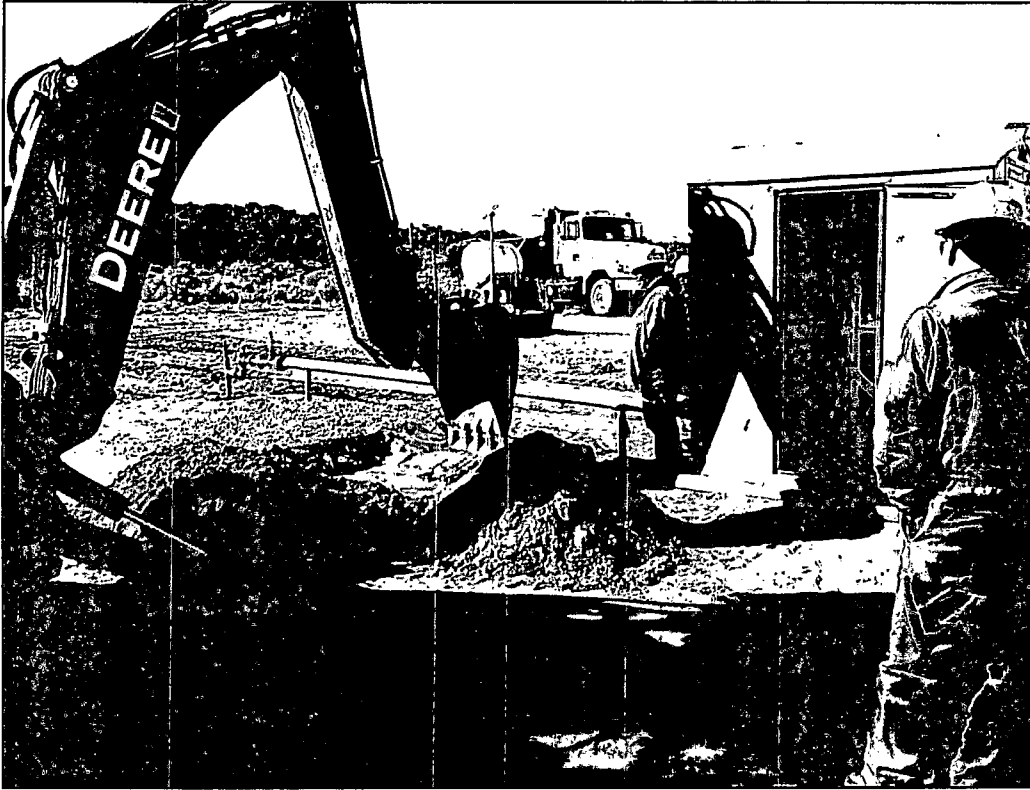
Photo 3: Excavation contractor removing soil at depth from the southwest corner of the meter house.
