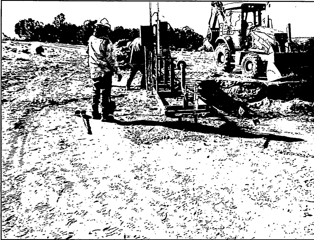
Photo 5: Photo of backfilling activities around the meter skid using imported material.
