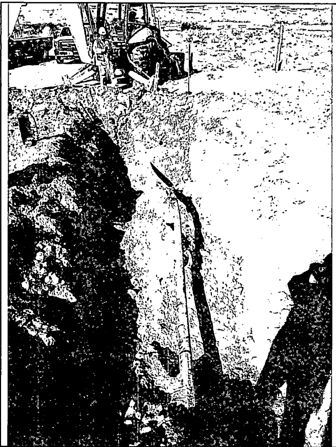
1.) Early stages of excavation facing to the west. Showing where the pipeline had been struck by something in the past (source of leak).
