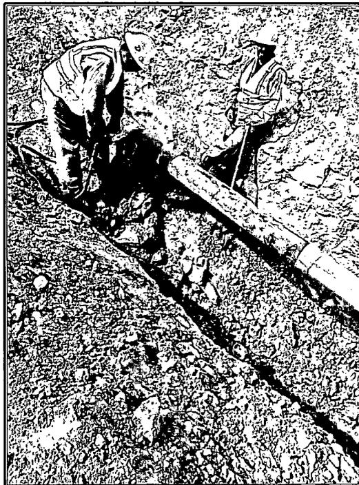
Photo 4: View of Lateral 2C-6 pipeline excavation continuing through the bedrock base using an air powered jackhammer.
