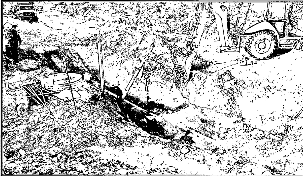
Photo 1: Beginning of excavation at the Lateral L-14A pipeline release at a depth of approximately 4' bgs. Strong odor present
