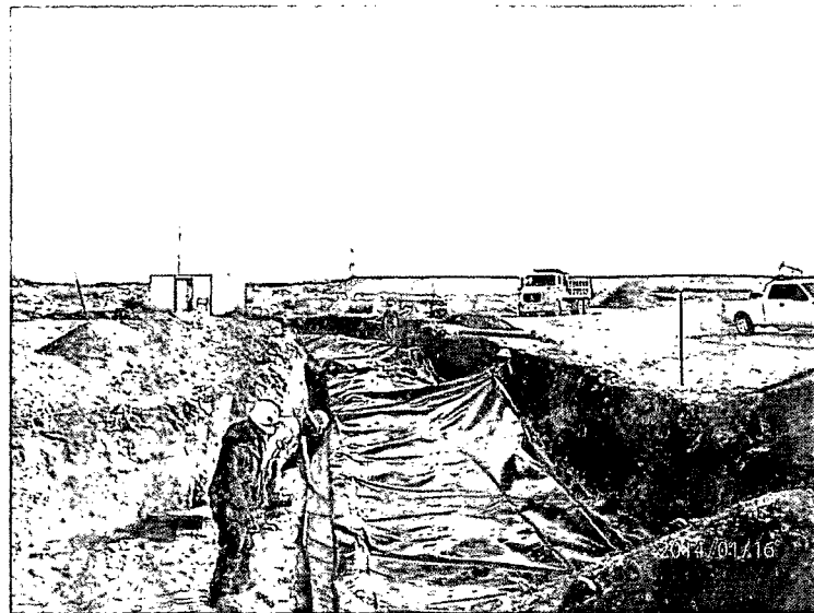
Installing 20-mil poly liner, facing east
