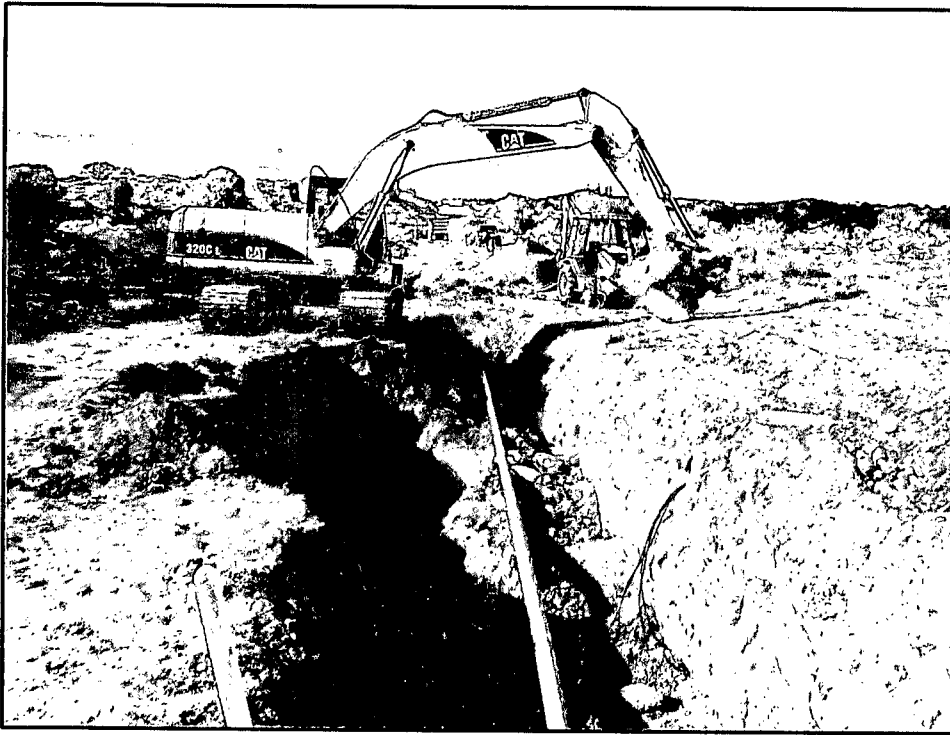
Photo 5: Continued excavation of the Ludwick LS #18 pipeline beyond the reach of 12 feet by a rubber-tired backhoe.
