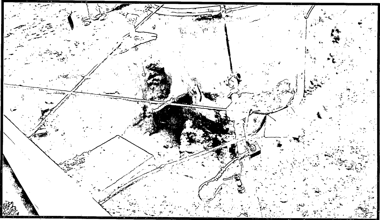
Photo 6: Pipe fully exposed, leak located in pipe center right of image. Black and grey contaminated soil visible around base of BGT.
