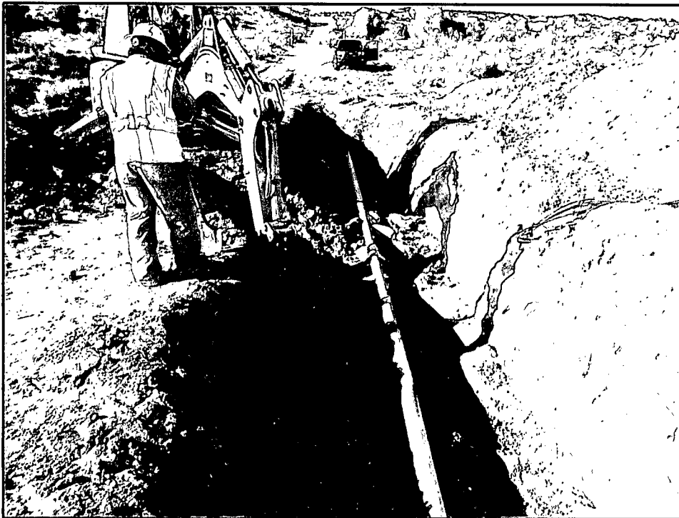
Photo 4: Preliminary remediation excavation following completion of the repairs to the Ludwick LS #18 pipeline.
